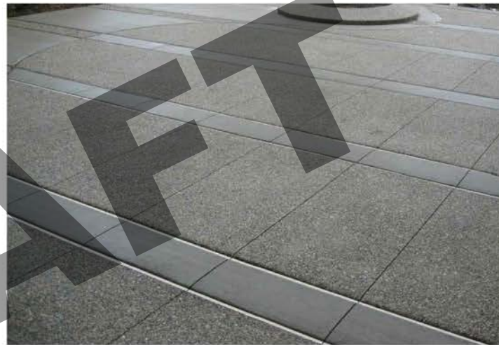
Washed aggregate in concrete paving
