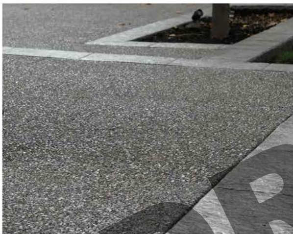
Washed aggregate in concrete paving
