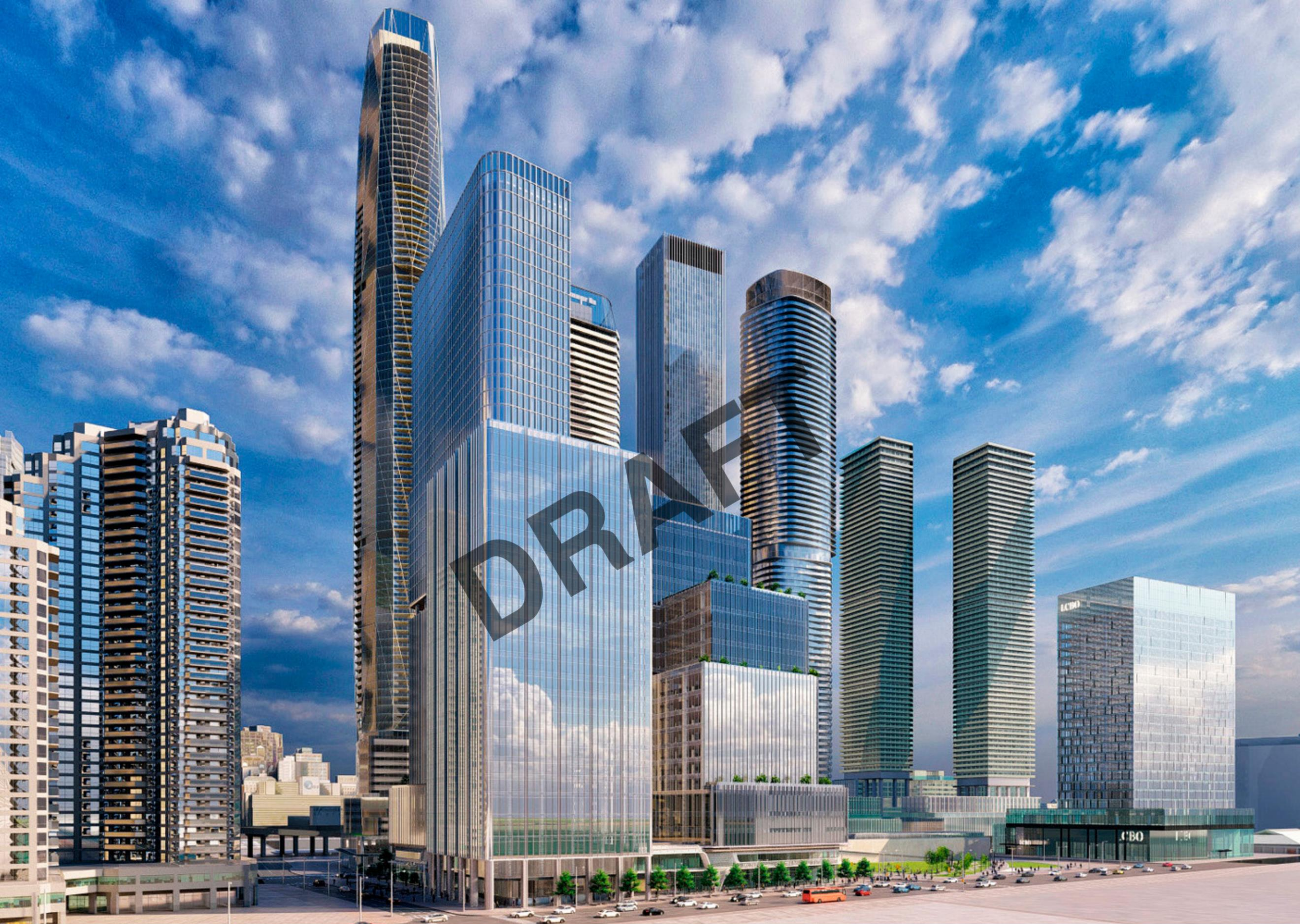
Queens Quay Looking North
