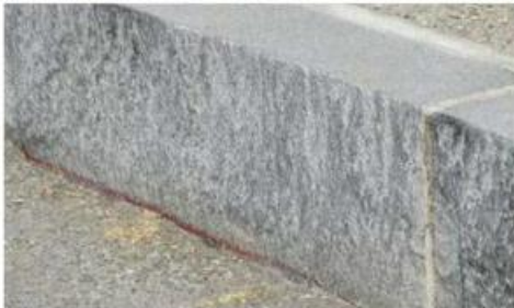
Figure 3.13 Granite curb example
