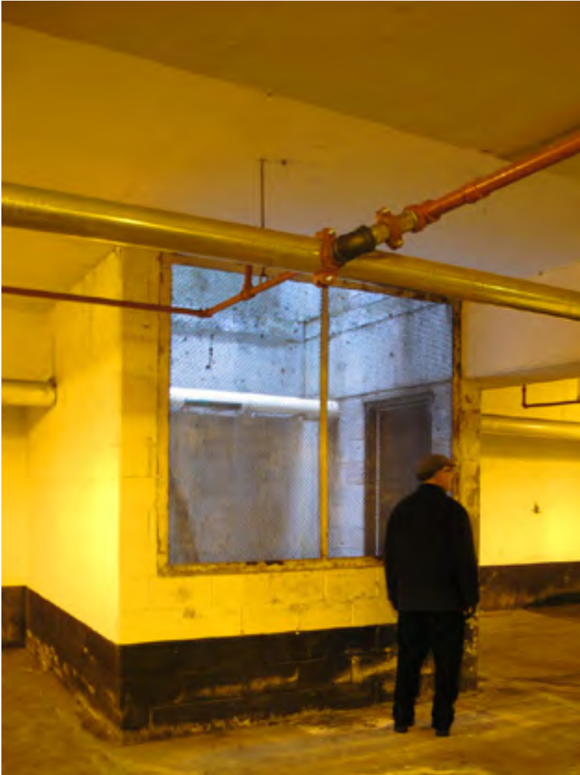
Daylight radically contrasts with both the intensity and the color rendition of standard parking garage lighting
