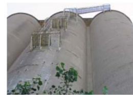
(top) The 'Image Mill' video projection installation to celebrate Quebec City's 400th year involved dazzling projections on industrial buildings and structures in the harbour. (above) Existing Victory Soya silos
