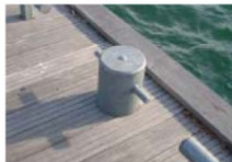
Galvanized steel mooring
