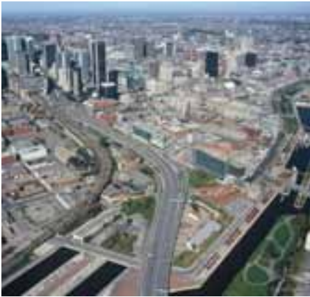
The Bonaventure Expressway enters downtown Montreal from the east; Peel Basin and Lachine Canal are in the foreground.
