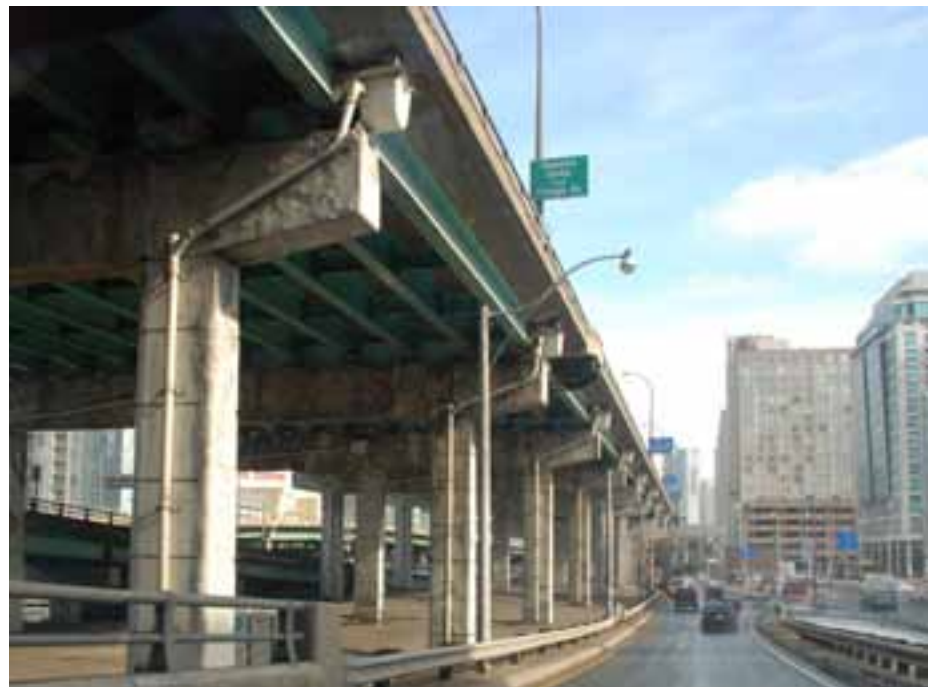
Gardiner Expressway in downtown Toronto.
