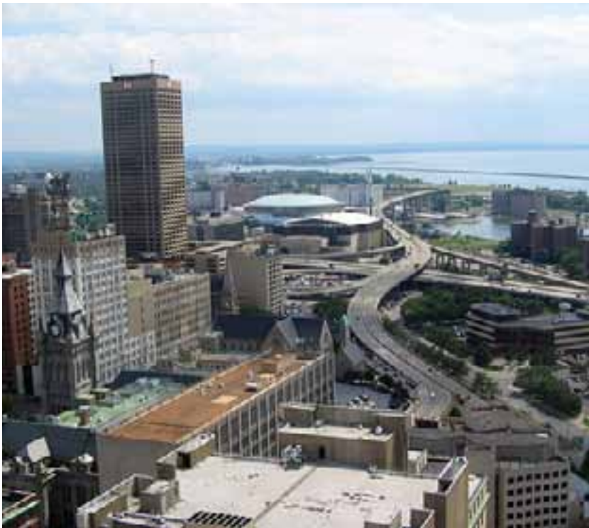
View of Skyway facing south.
