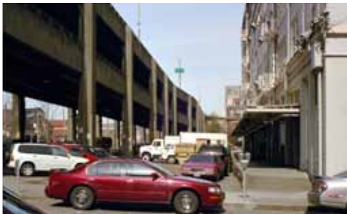
Existing condition under the Viaduct.
