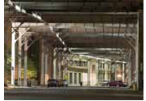
Existing condition on K Street under the elevated structure.
