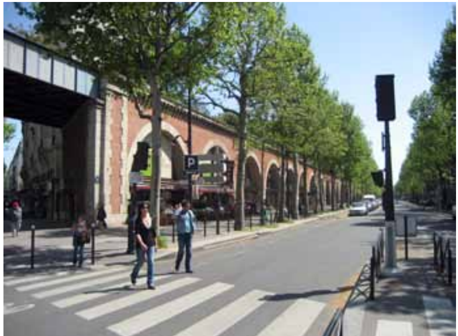
The archways under the viaduct provide space for artist studios, workshops, and restaurants.
