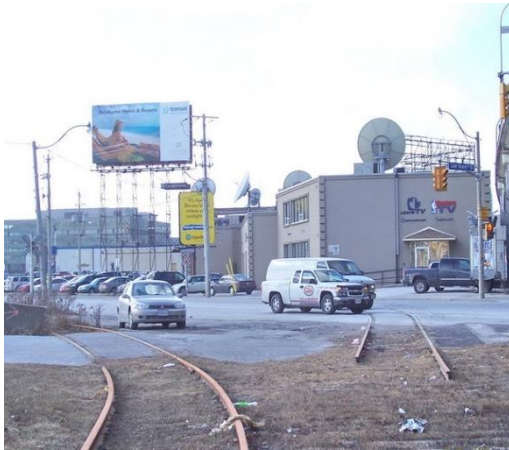
Abandoned Spur line curves south beside Parliament Street. Turnout has been decommissioned and the Track crossing Parliament Street is still in place.
