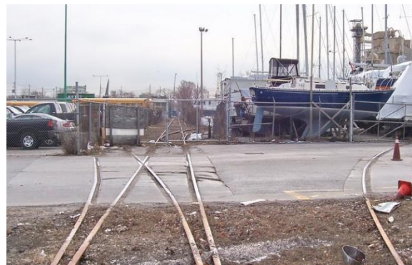
Lead track crossing Commissioners Street.
