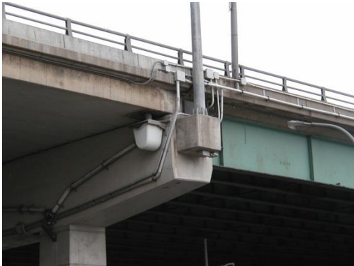
Gardiner Deck at Jarvis Street
