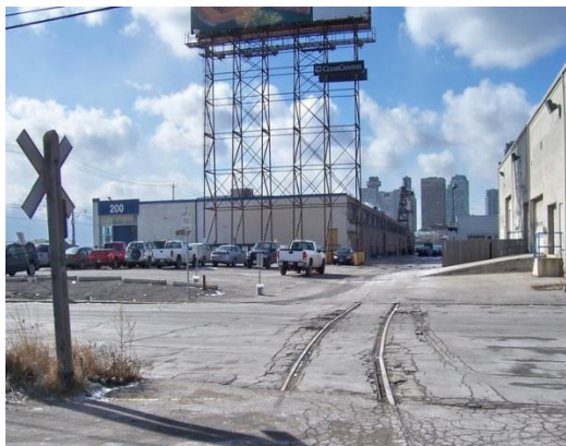
Spur line that crosses Parliament Street, Small Street, and Bonnycastle Street. However, the portion of track beside the adjacent Industries has been paved over for parking.
