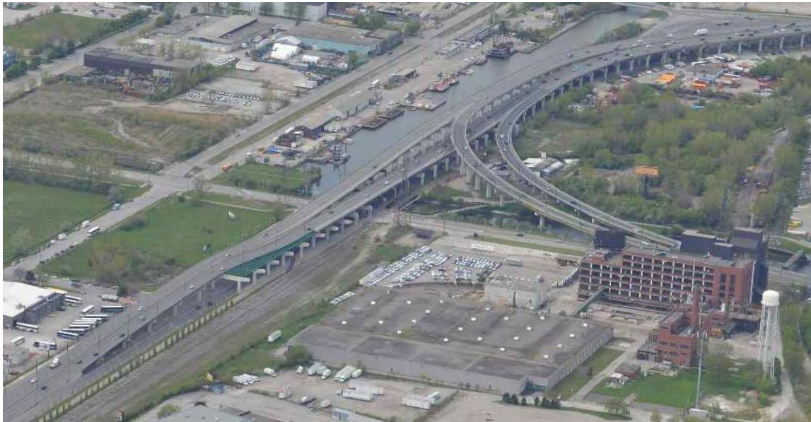
Eastern Terminus of the Gardiner Expressway and DVP Ramps looking southwest
