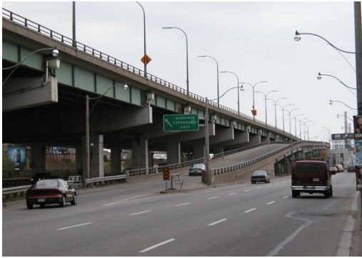
Light Pole and Parapet Arrangement
