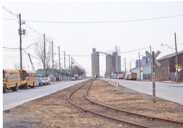
One leg of the lead track along the median on Villiers Street toward Cherry Street.
