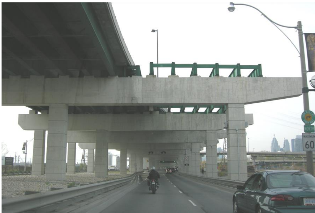
Gardiner Expressway structure east of the Don River with Lake Shore Boulevard below – looking west
