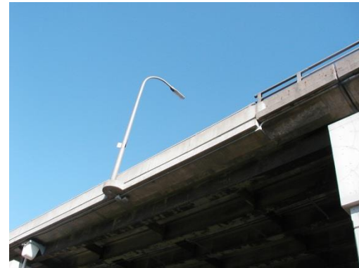
Gardiner Deck at Don Valley Parkway
