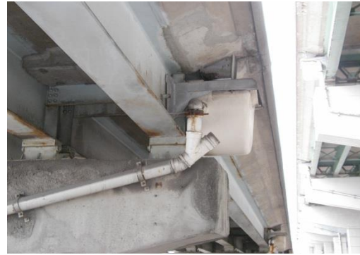
Typical Hopper Attached to Steel Girder
