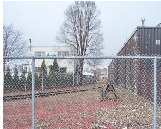
End of Track at Polson Street
