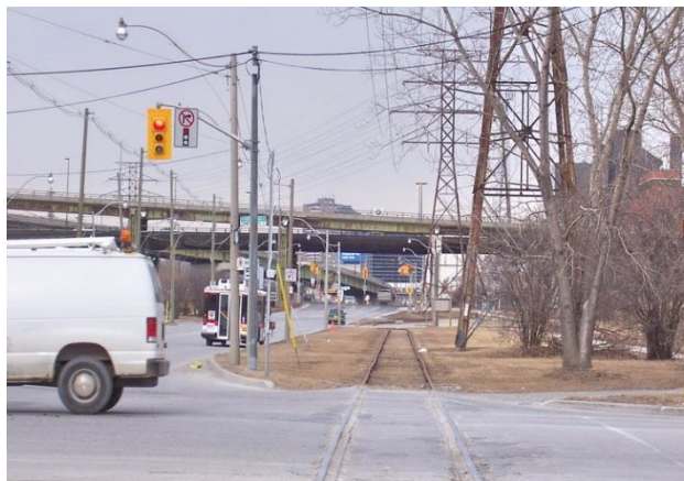
Lead track ends South of Commissioners Street.
