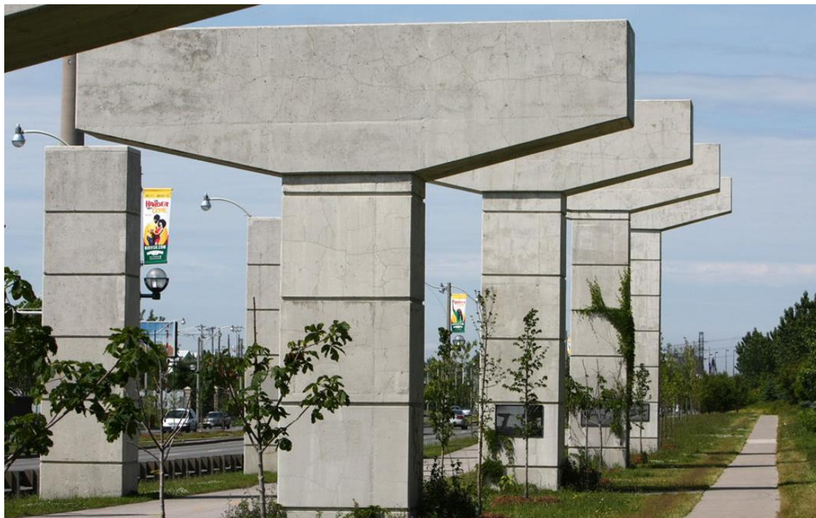
Lake Shore Boulevard Commemorative Art Treatment with Bike Path – just west of Leslie Street looking west
