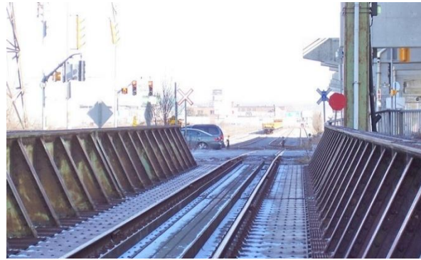
Steel Bridge over the Don River.
