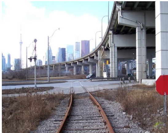
Railway spur line crossing Cherry Street and Lake Shore Boulevard (looking west on the south side of the Gardiner)
