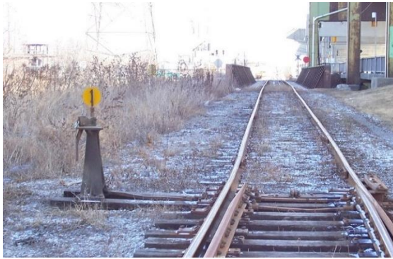
Harbour track heads eastward crossing over the Don River and Don Roadway and entering Keating yard.
