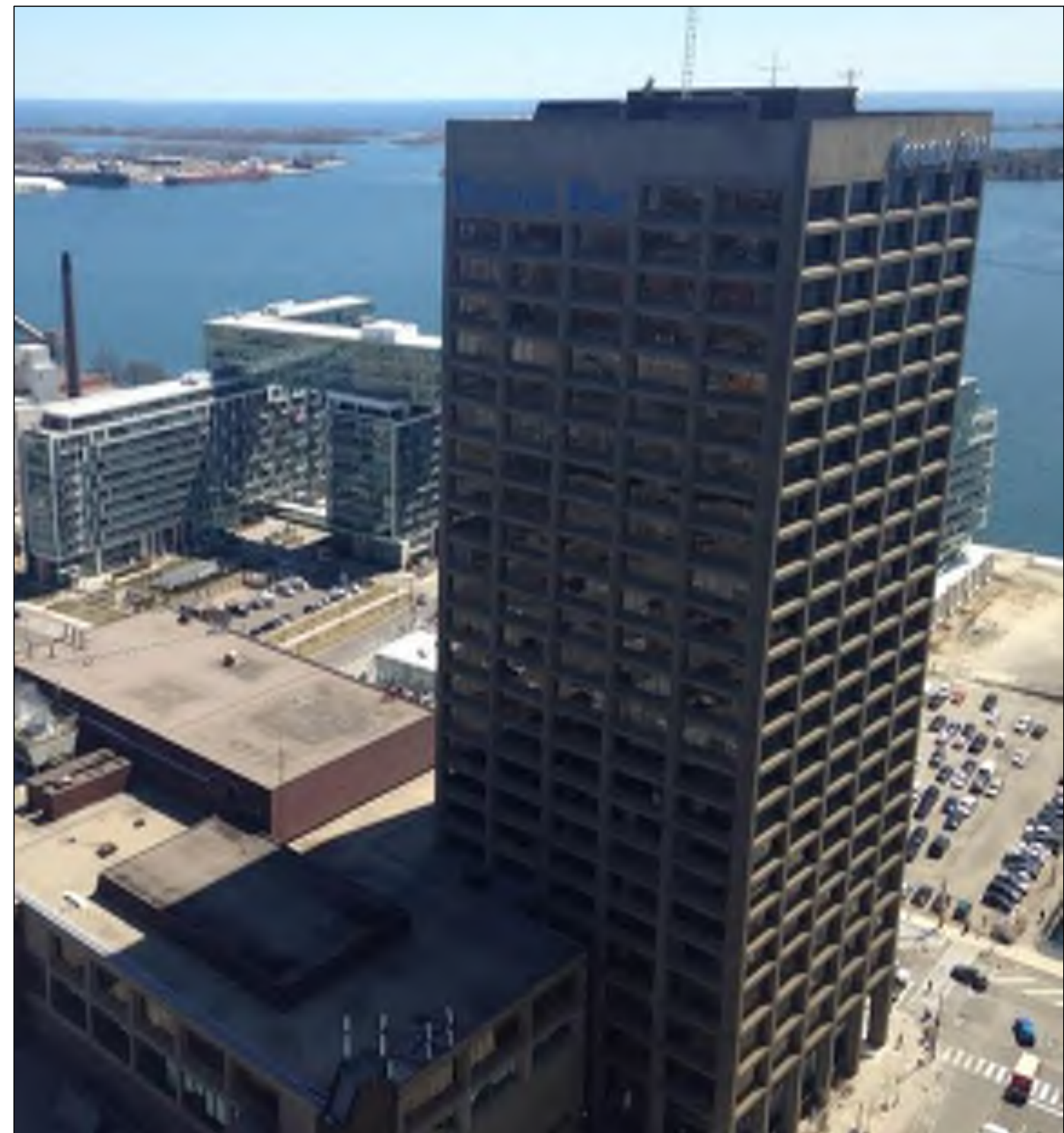
Toronto Star Building, looking southeast
