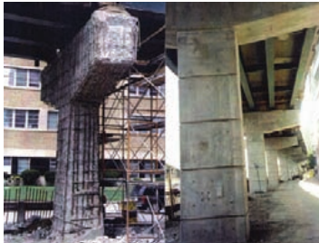
Some corroded concrete columns have been repaired.
