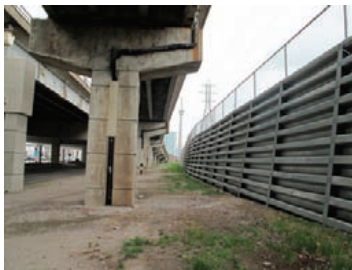
The elevated structure is a barrier.
