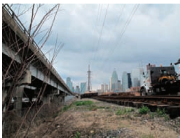
The railroad viaduct and easement pose a second waterfront barrier.
