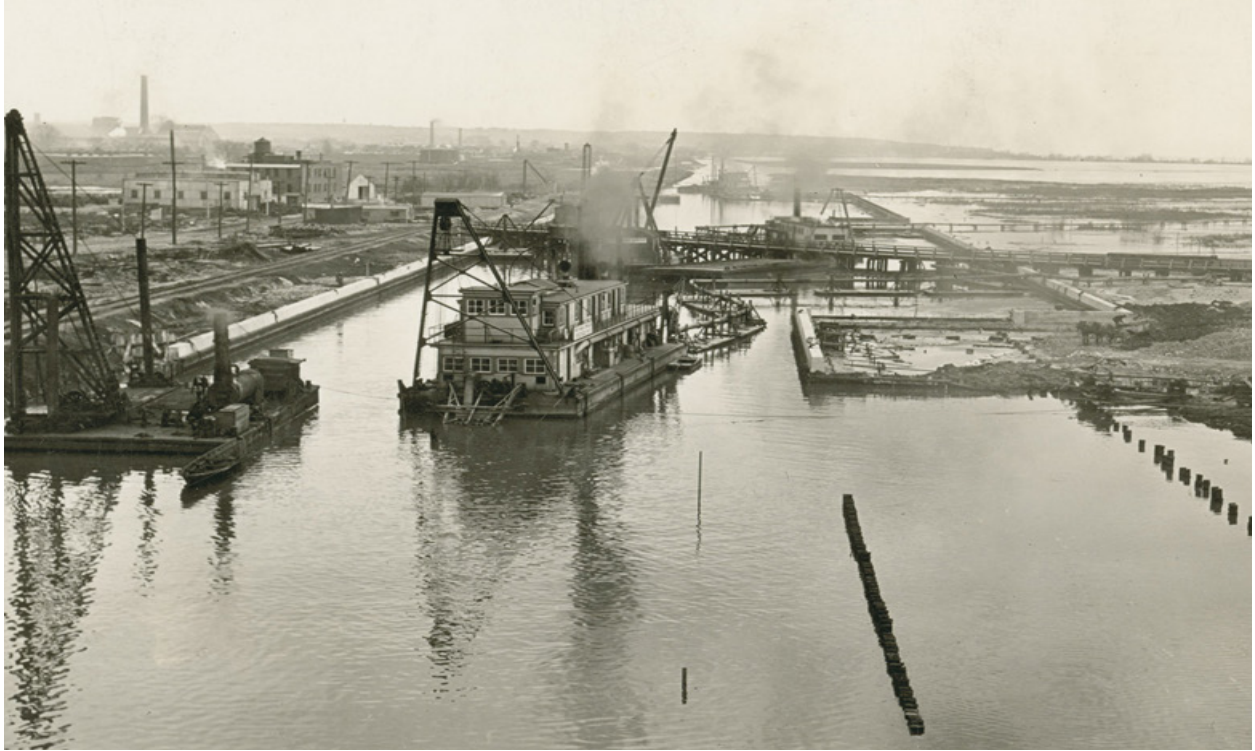
Looking east during construction of the Keating Channel in 1914. Source: City of Toronto Archives
