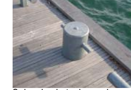
Galvanized steel mooring
