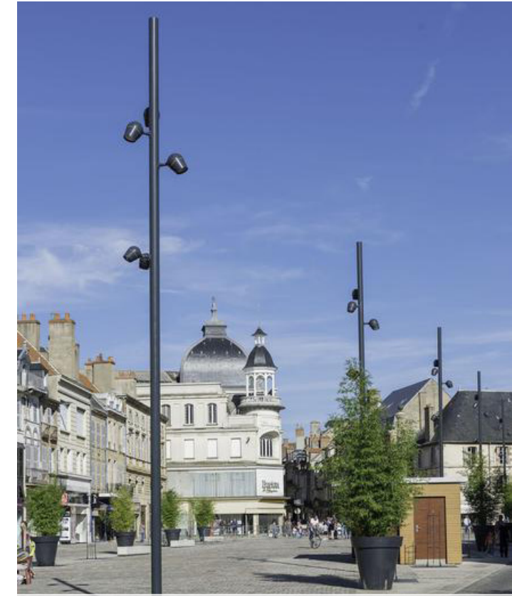
Tall Mast Lighting
