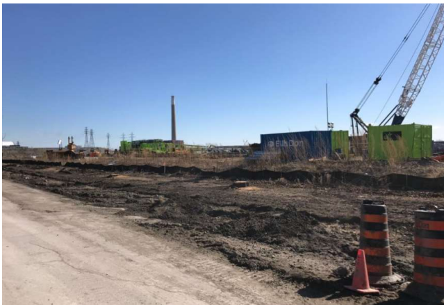
Figure 3 Commissioners St - Site Preparation
