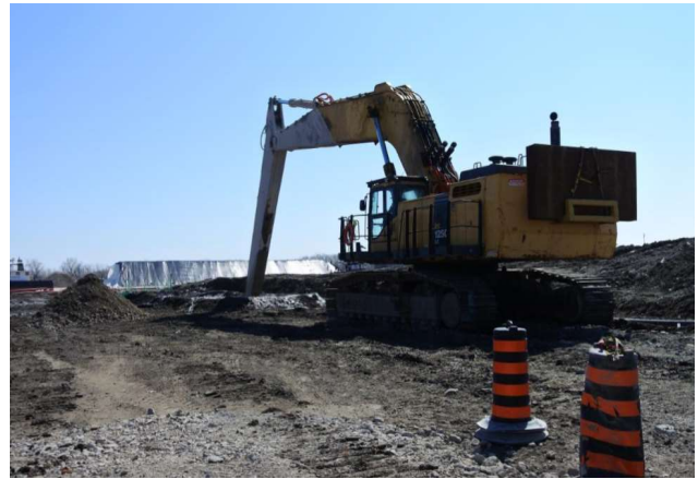
Figure 2 River Valley - Excavation Works in Slurry Wall
