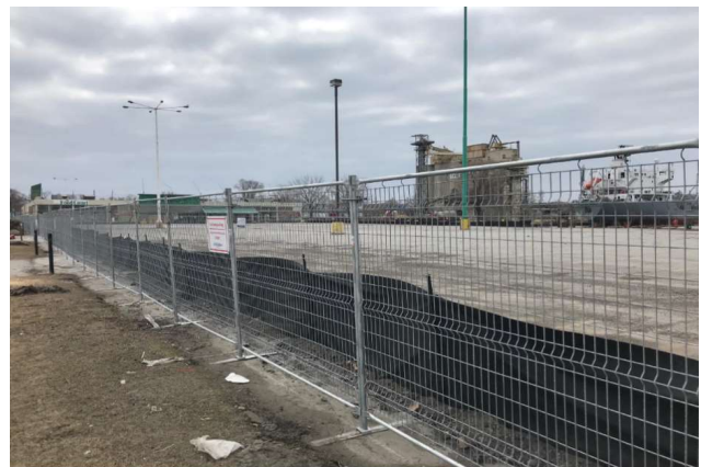
Figure 6 Cherry St Bridge South - Site Preparation
