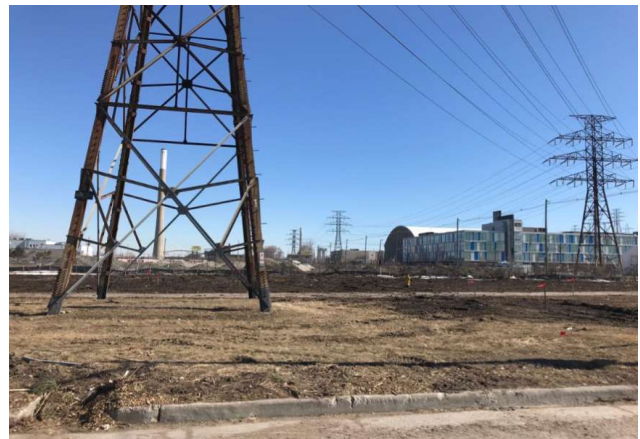
Figure 4 Hydro One - Tree Cutting & Site Preparation
