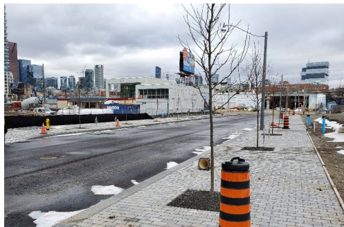
Streetlights and trees installed on Merchants Wharf looking north
