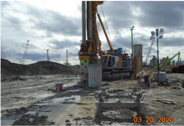
Figure 1 Cut-off Wall Phase 1 - Drilling Holes for Pile Installation
