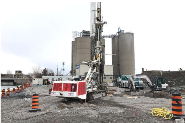
Figure 5 Cherry St Bridge North - South Abutment Remediation of Foundation Works
