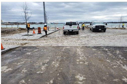
Concrete roadway pavers installed at St B and C looking south
