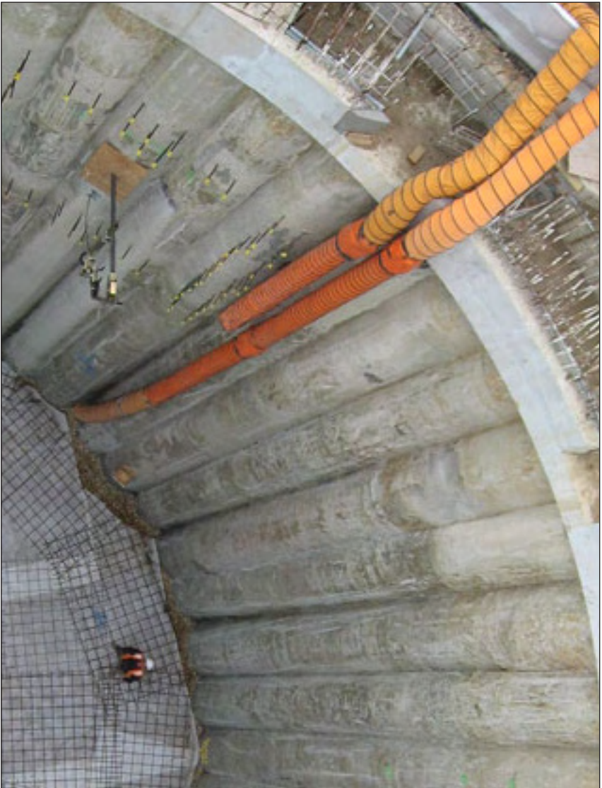
Secant Wall Construction
