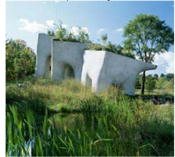
elevated wetland by noel harding
