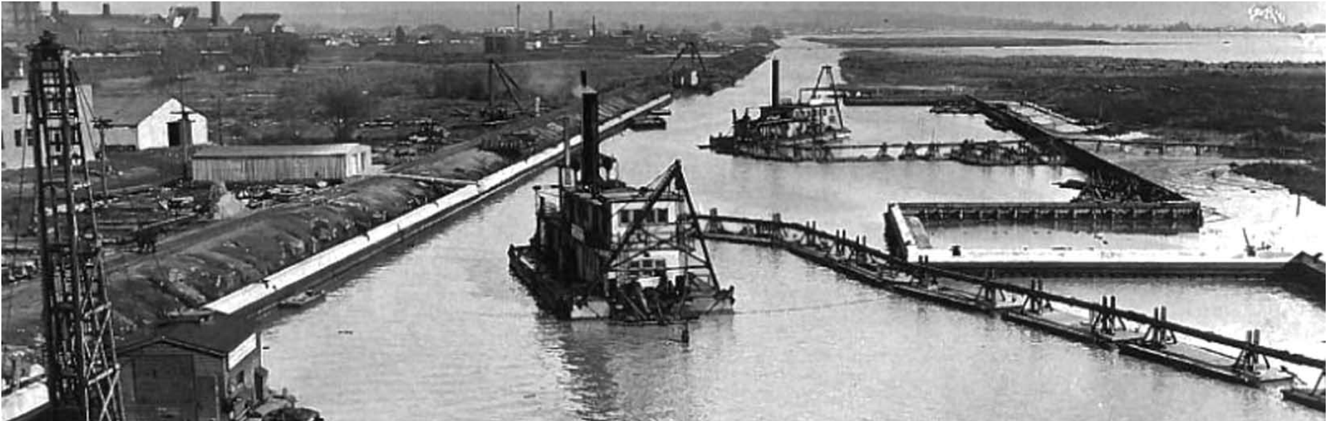
Building the Channel
