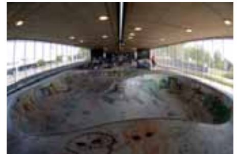
Cladding and lighting on the highway columns makes the space more inviting; the skate-park generates amble activity.
