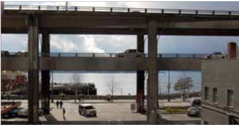
Parking is a common use under the Viaduct.
