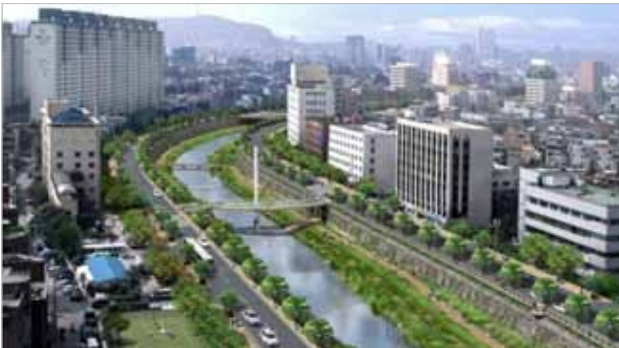
The Cheonggyecheon Expressway contributed to declining property values and population loss in Seoul's downtown before it was replaced by a linear park.
