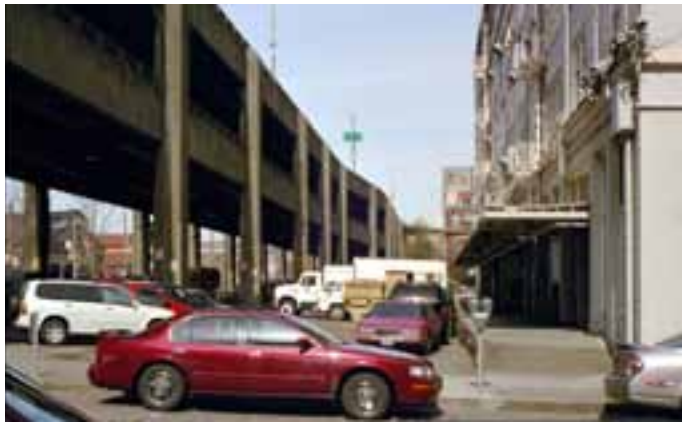
Existing condition under the Viaduct.
