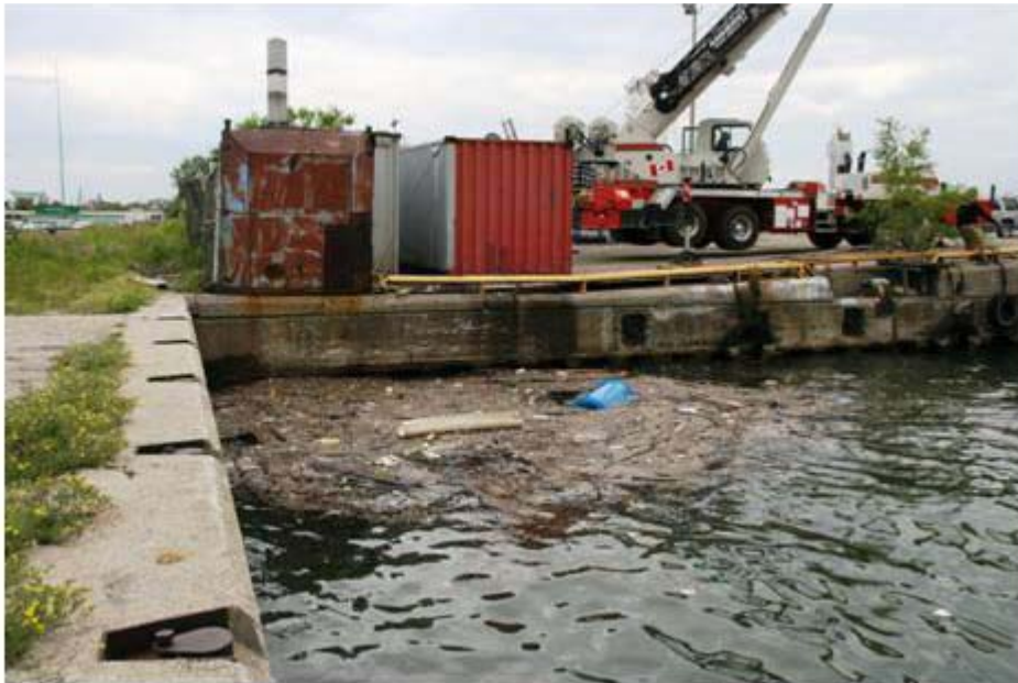
Commissioners Street Storm Outfall
