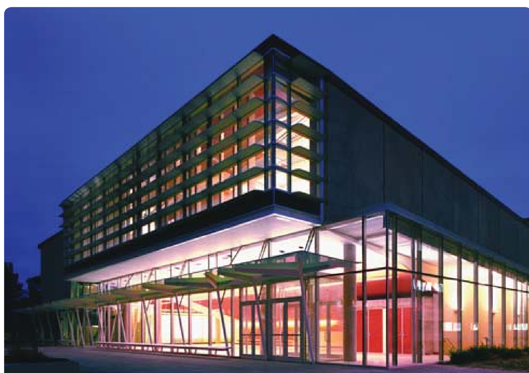
York University Computer Science Facility in Toronto is considered the most energy efficient green building built in a cold-climate location in Canada.
