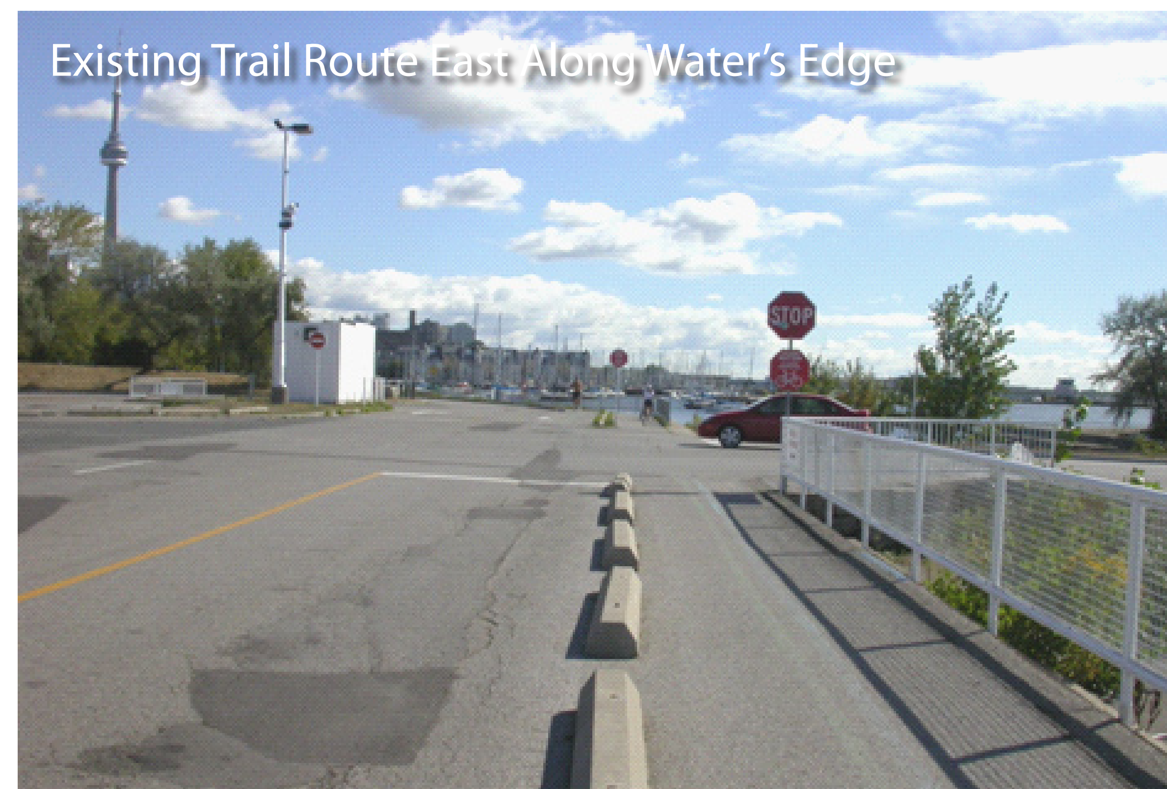
Multiple users + constrained trail = spillover into vehicular lanes
