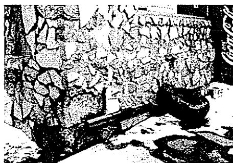
View of exposure of the heavy cut limestone foundation of the 589 King Street East building.
