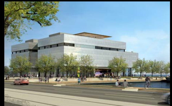
January 21, 2008 Addition of 8 th Floor and canopy
