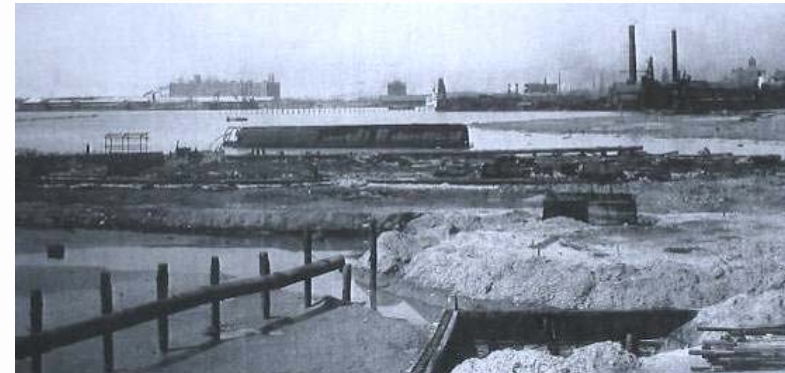
View of the derelict ship from Sherbourne Street, May 1927. Stripping of plates from the upper hull is underway
