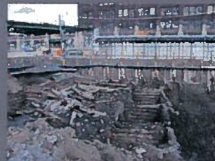
1850's crib work uncovered at Queens Wharf
