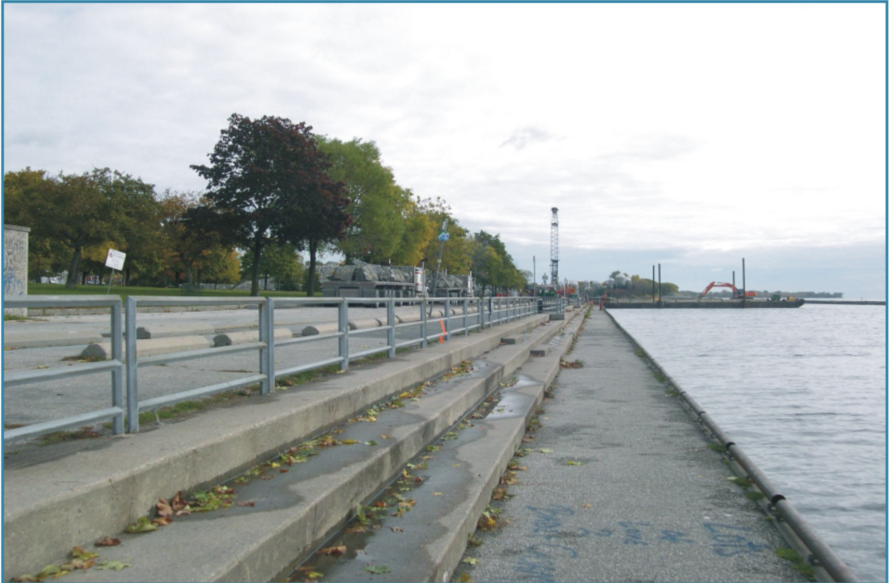
PROMENADE - TYPICAL CONDITION “BEFORE”
