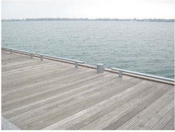
"TREX" RECLAIMED WOOD AND PLASTIC BOARDWALK. LOW GALVANISED METAL RAILING.
