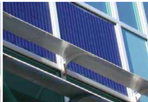
Solar paneled facades and sun shades on south building faces
