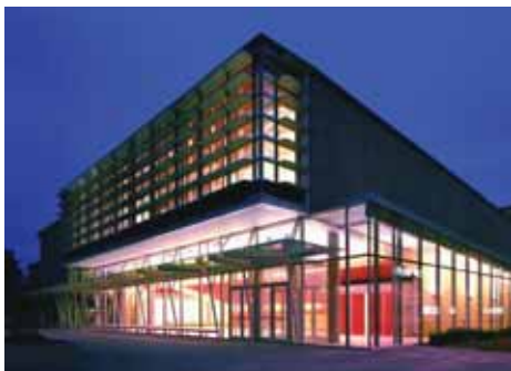
York University Computer Science Facility in Toronto is considered the most energy efficient green building built in a cold-climate location in Canada.
