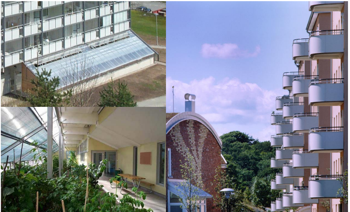
Figure S6 A Swedish Reference Example of Sustainable Building Design: Gårdsten in Gothenburg and Mälarstrand in Stockholm
