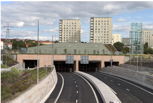
Figure 2:9 The Southern Link – a newly inaugurated Highway Tunnel in Stockholm.
