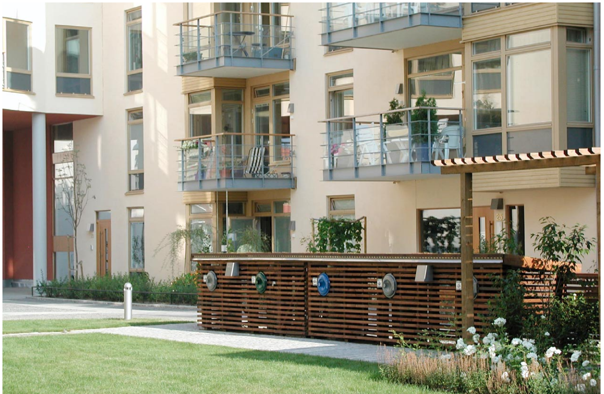
Figure 3:14 An Example of a CVC-system. The Inlets of the System are carefully designed as part of the Urban Environment in Hammarby Sjöstad in Stockholm.
