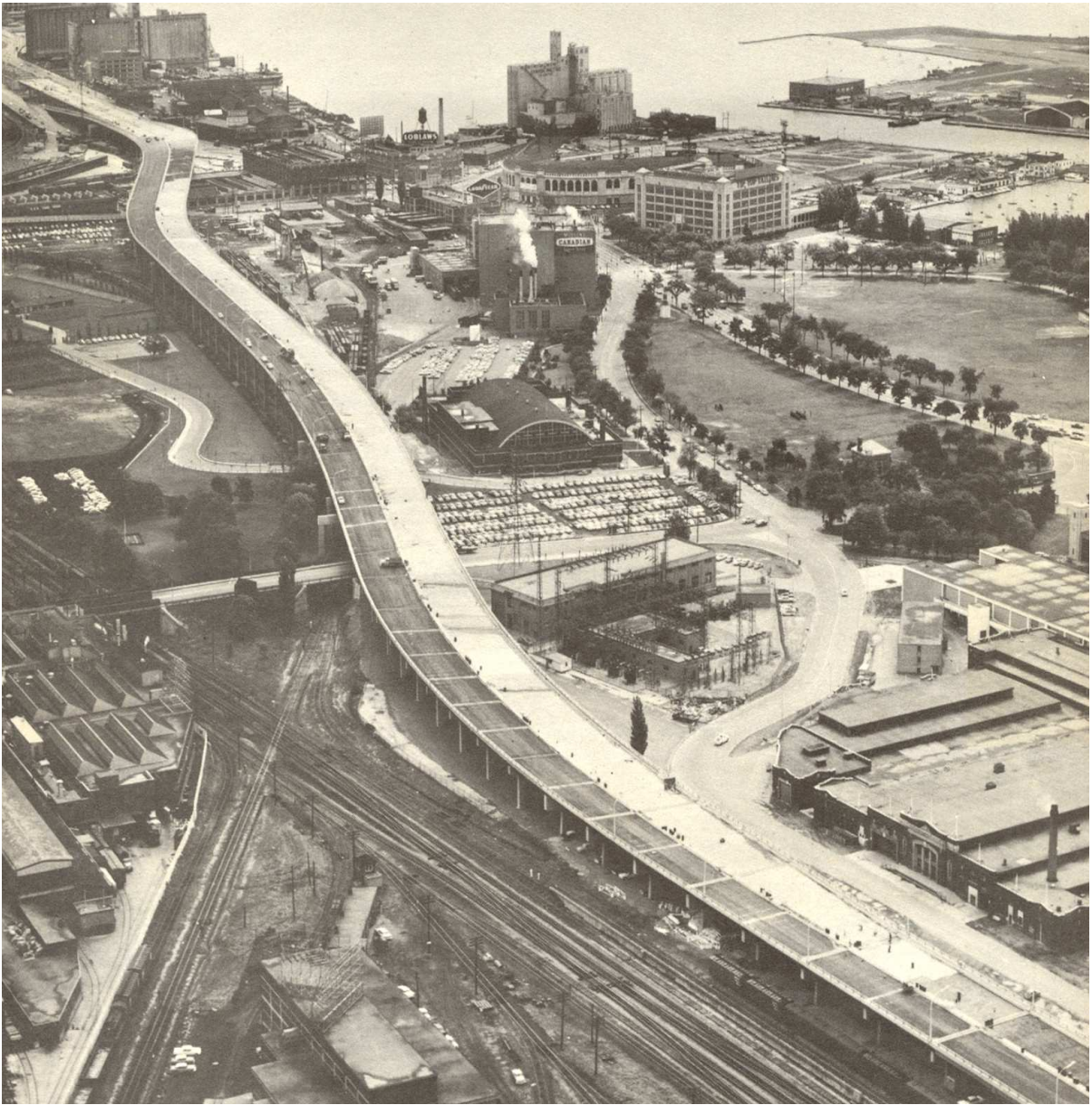
Gardiner Expressway Under Construction, 1960's
