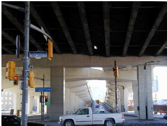
Some Ramps are Impediments to Accessing the Lake Front.
