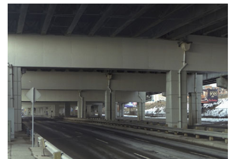
Figure: Existing view of Gardiner at Parliament Street
