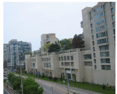
Figure: Back of King's Landing facing the Gardiner/Lake Shore Corridor
