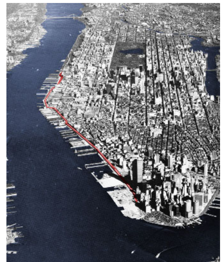
Figure: Westside Highway, New York
