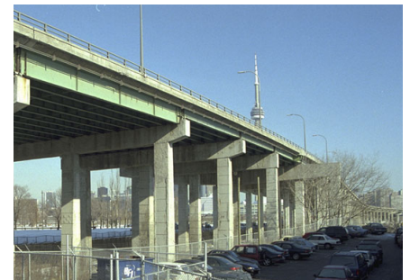
Figure: Existing view of Gardiner at Fort York
