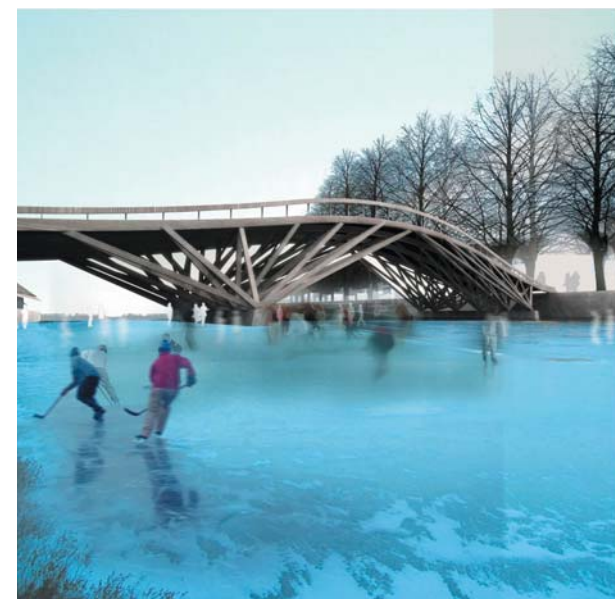
TIMBER PEDESTRIAN BRIDGE CROSSING OVER YONGE SLIP TO THE NEW FERRY TERMINAL
