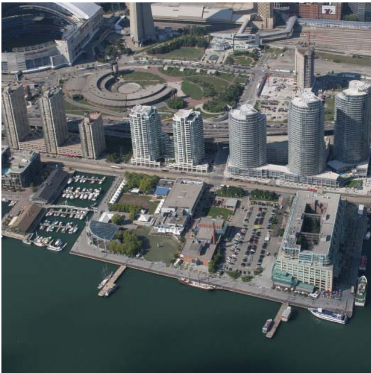
York Quay and Simcoe Slip looking north
