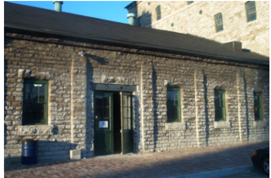
Fermenting Room entrance, Distillery District
