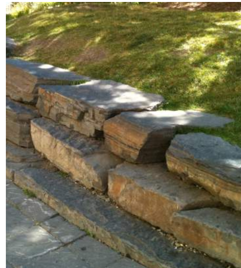
Armourstone seat wall
