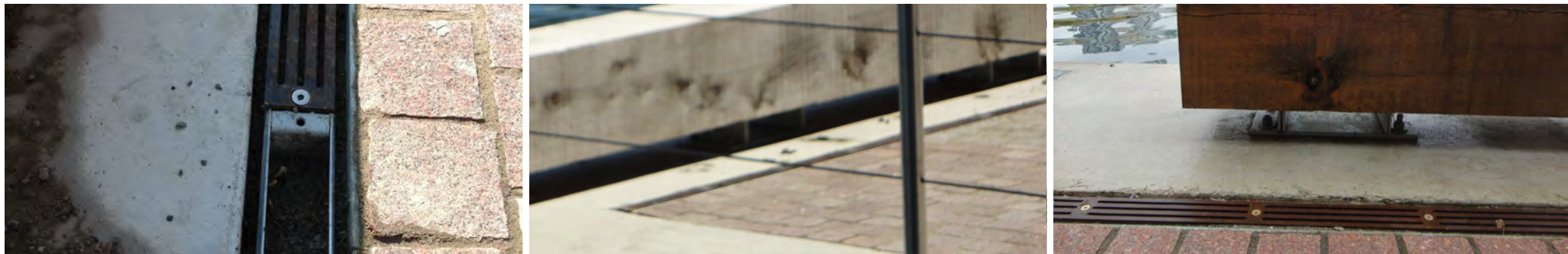
the use of a continuous trench drain on the side of the promenade (tree line) (reference of Portland Slip Water's Edge Promenade)
