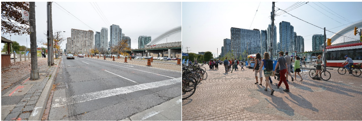
Left: Looking west on the south side of Queens Quay in 2012 before construction began. Right: Looking west from the same location after construction was completed in 2015.
