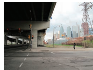
View of Lower Don Lands and Gardiner Expressway from the south-east.
