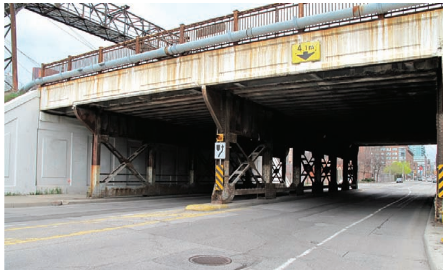
There are few pedestrian and vehicular connections under the viaduct.
