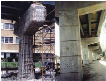
Some corroded concrete columns have been repaired.
