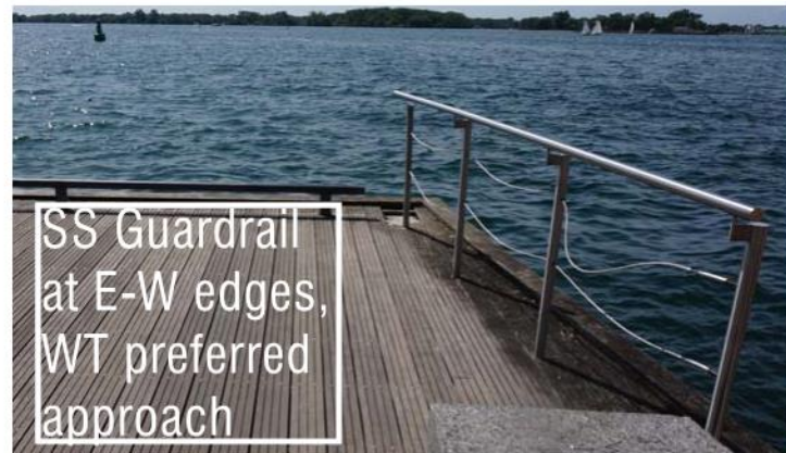
York Quay and Police Basin Boardwalks - Toe Rail with Stainless Steel Guardrail
