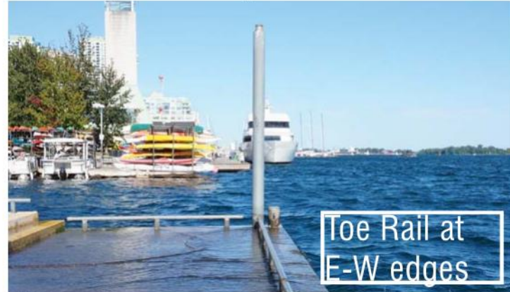
HTO Park Boardwalk - Toe Rail with Navigational light on steel pile
