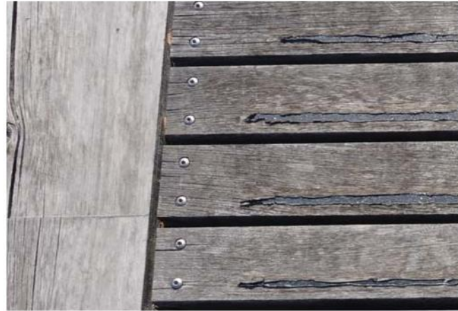
Reference: countersunk tamper-proof screws, existing Wave Deck
