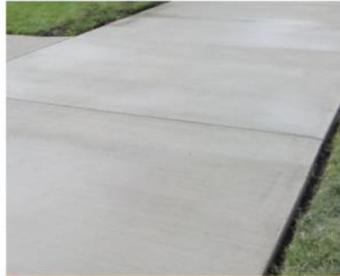
CIP Concrete Pavement
