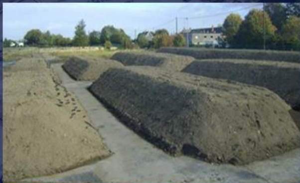
Soil Treatment for Soil Exceeding Environmental Thresholds
