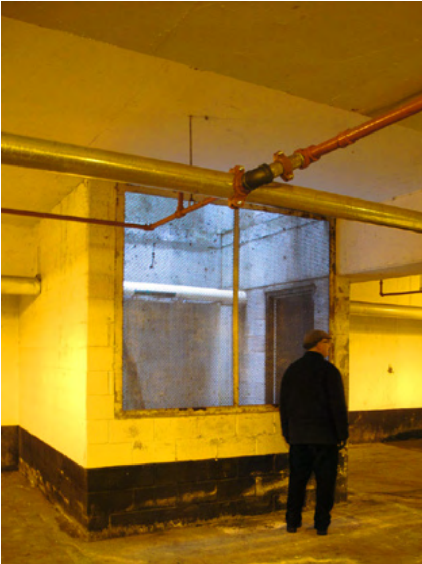
Daylight radically contrasts both the intensity and the color rendition of lighting standards for parking garages
