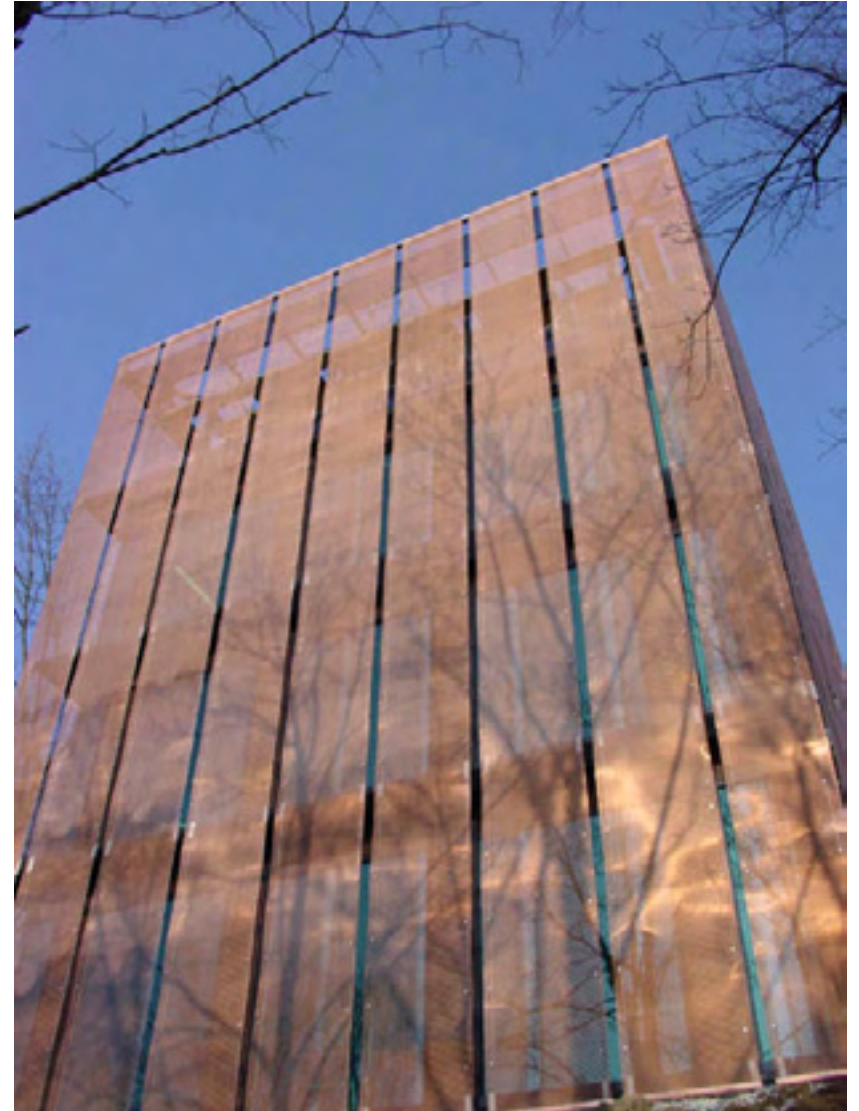
Reflective perforated metal sheeting can be installed on tensioned stretcher bars as an affordable means for distributed daylight
