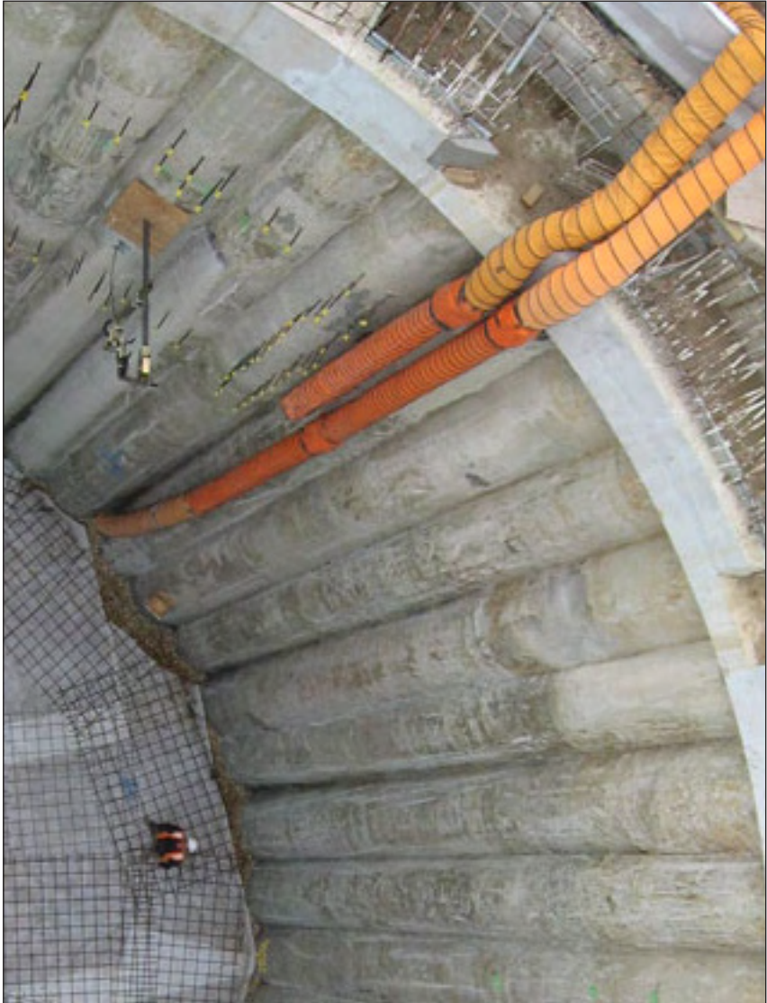
Secant Wall Construction
