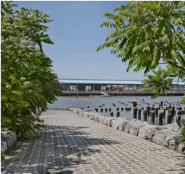
FIGURE 4-7: Example of armoured boat launch
