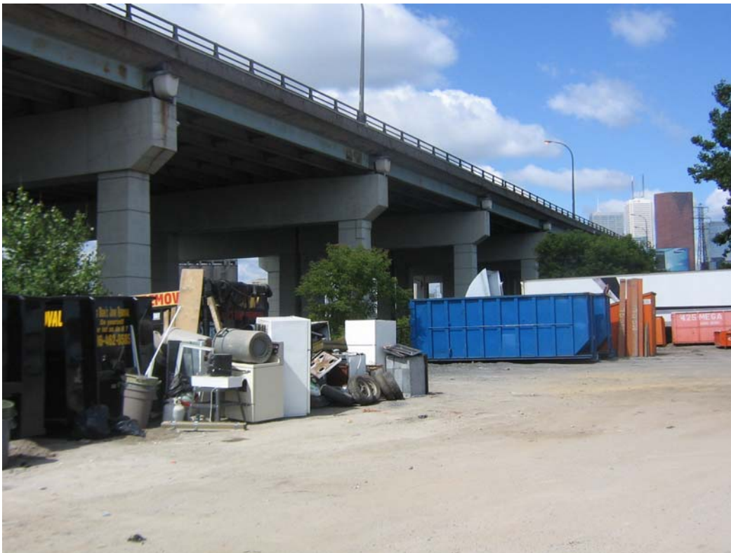
Photograph 2: Storage area on site at South side of Gardiner Expressway
