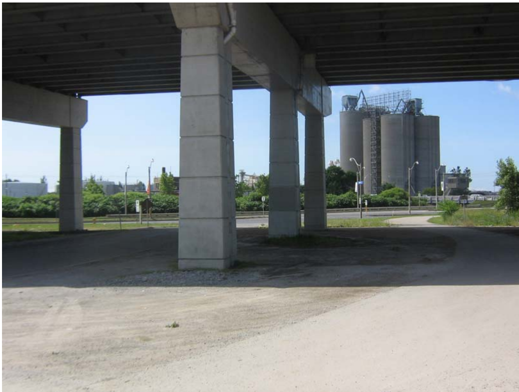
Photograph 8: View from South East of Site, looking South
