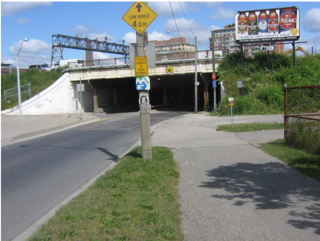
Photograph 6: At West edge of Site at Cherry Street, looking North
