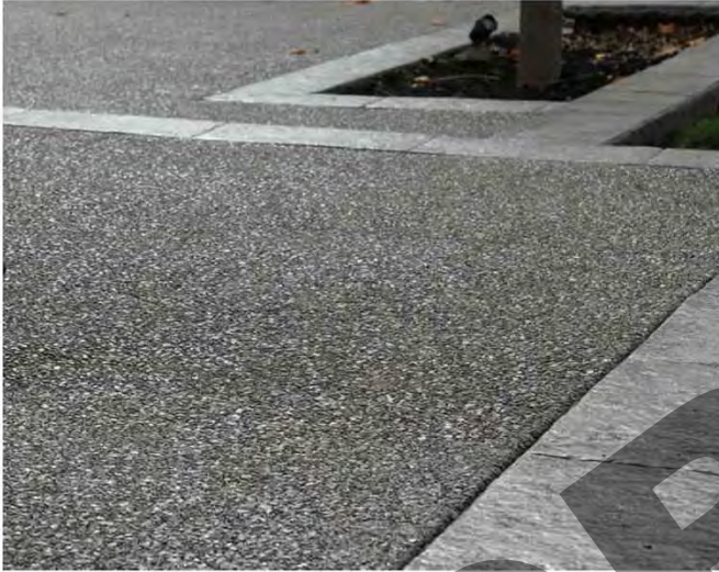
Washed aggregate in concrete paving
