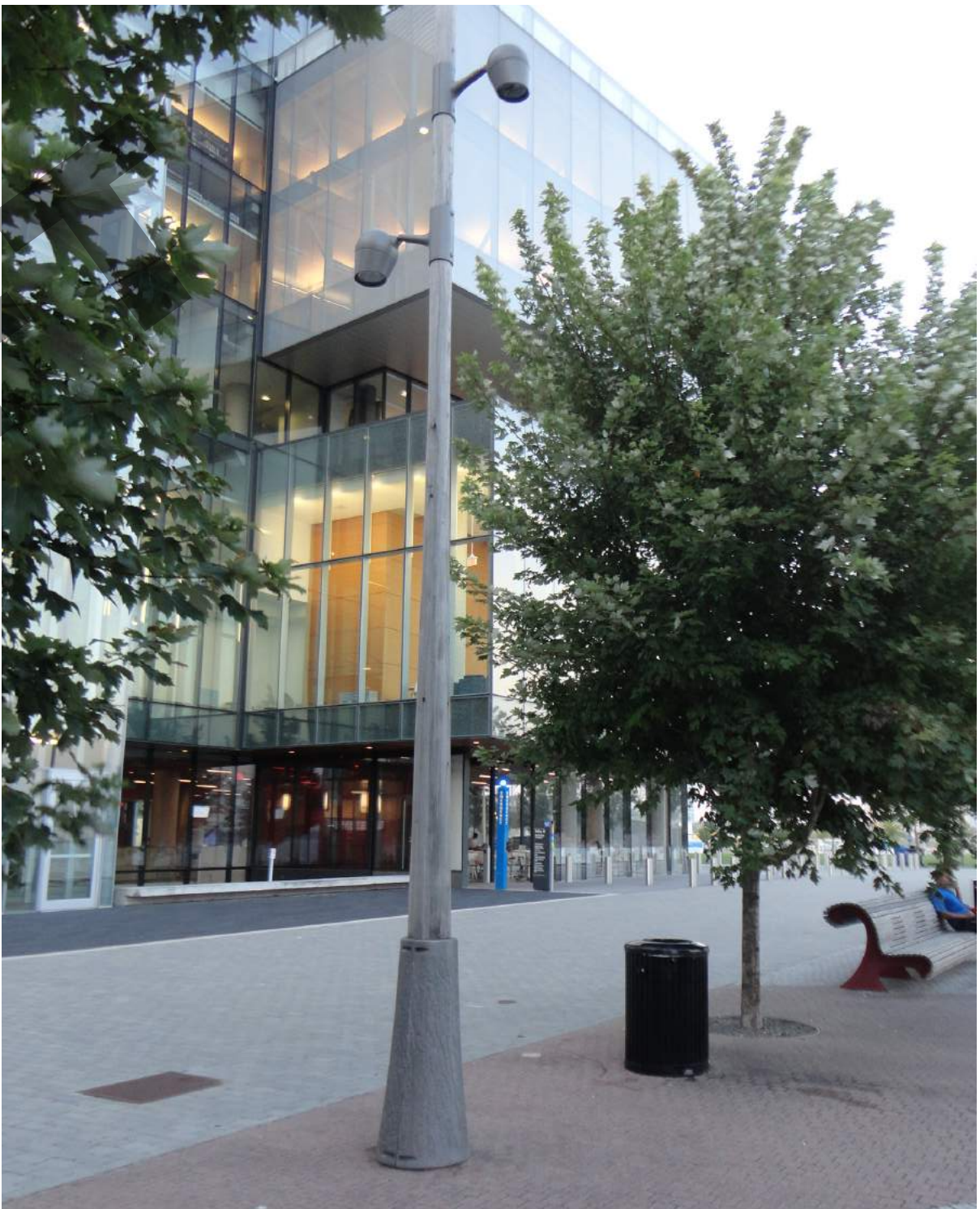
Waterfront Toronto signature light pole 6m high with Olivia light feature and shroud
