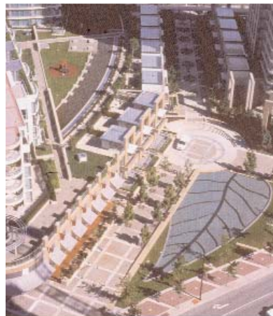
In Vancouver, townhouses surround a parking structure. Terraces and outdoor landscape space are built over the parking.
