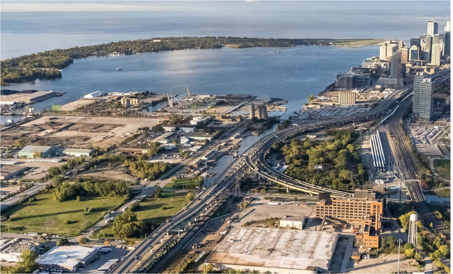
The Port Lands, where the Don meets Lake Ontario. Transformative earthworks and flood protection are now underway.
