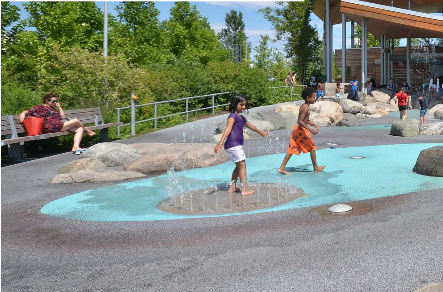
Corktown Common in the West Don Lands. The popular park is a carefully designed part of the flood-protection system around the Don River. Underground, a four-metre clay substructure reshapes the river’s floodplain, helping to safely direct flow south to the lake when water surges.
