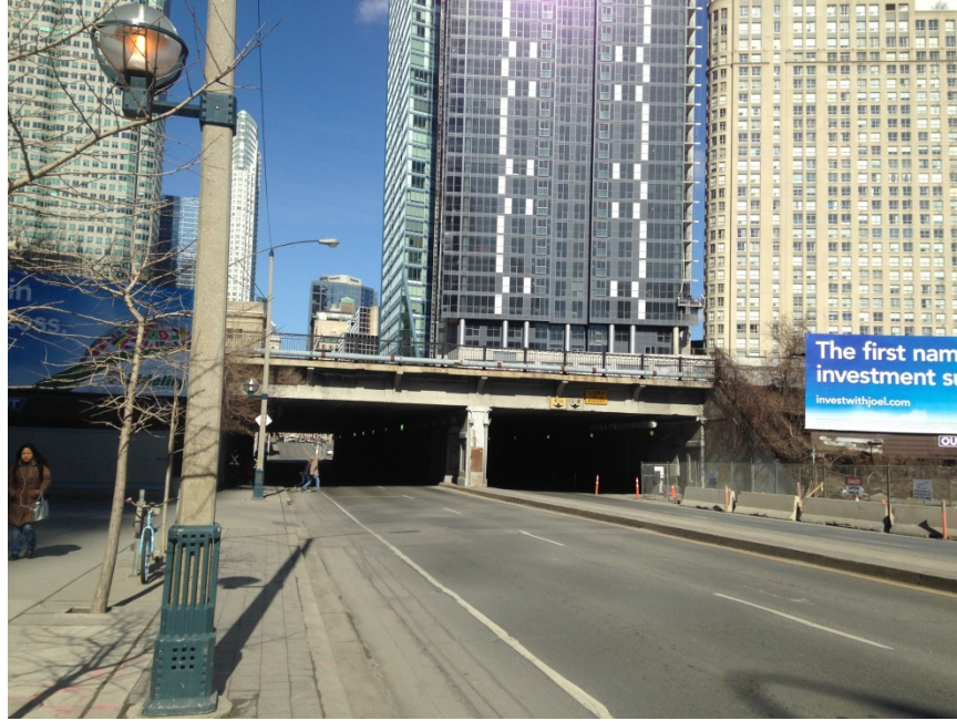
Photograph 11: View of Yonge Street, facing north
