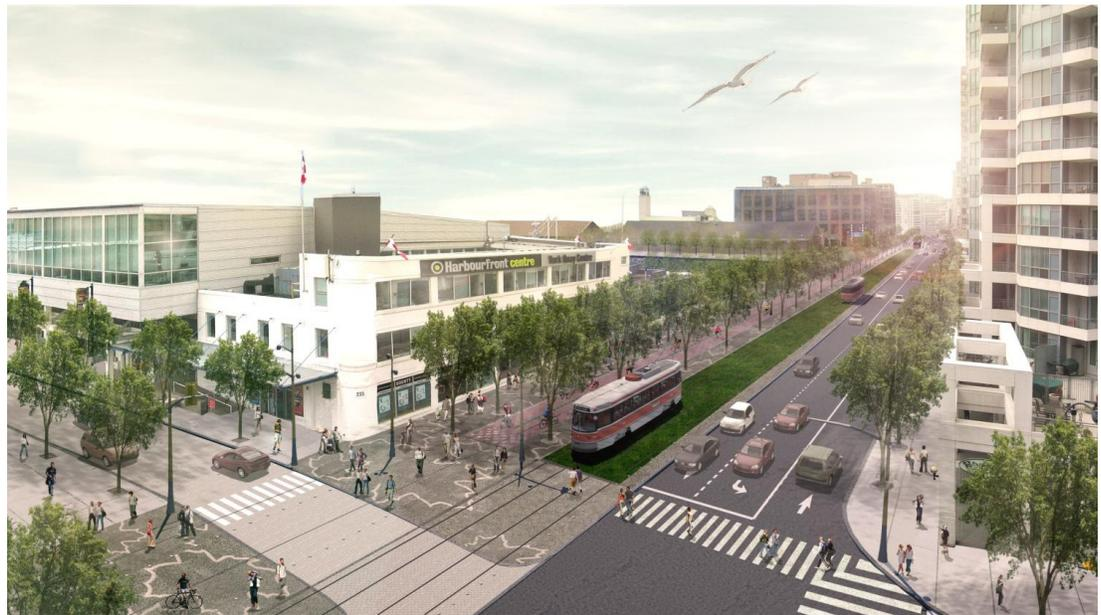
The Preferred Design, illustrated in Figure 9-1, Figure 9-2 and Figure 9-3, reconfigures the street by locating all traffic lanes north of the Light Rail Transit (LRT) right-of-way. Pedestrian and bicycle facilities would be provided on the southern side of Queens Quay where the existing eastbound lanes are located. Sidewalks would be provided on both sides of the street.
