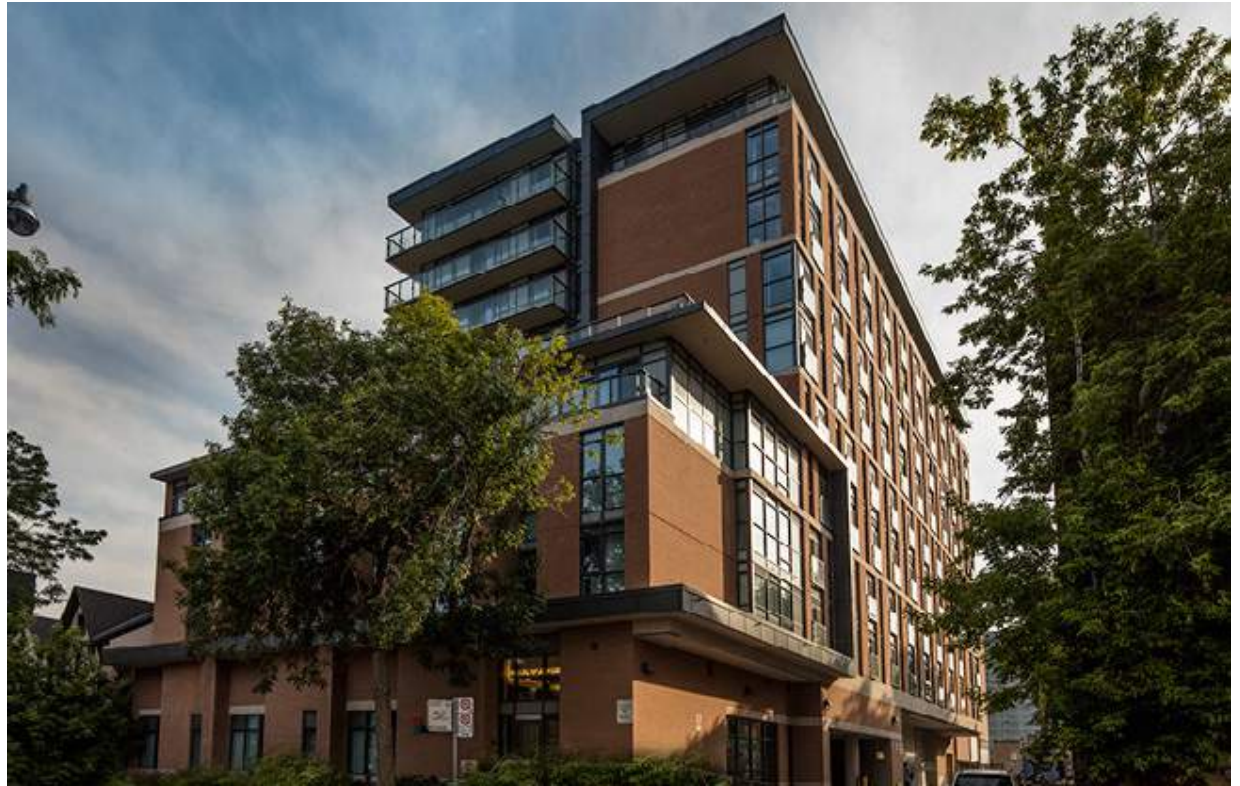
Figure 7.7 Low window-to-wall ratio and window wall system, 132 Berkeley Street, Toronto
