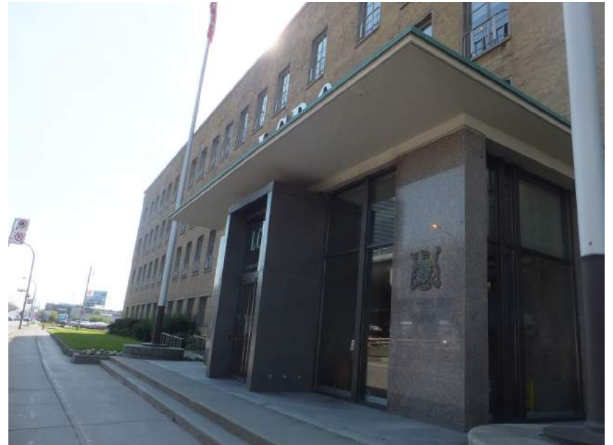
Figure 2.10 55 Lake Shore Boulevard LCBO Head Office, looking east from Freeland Street
