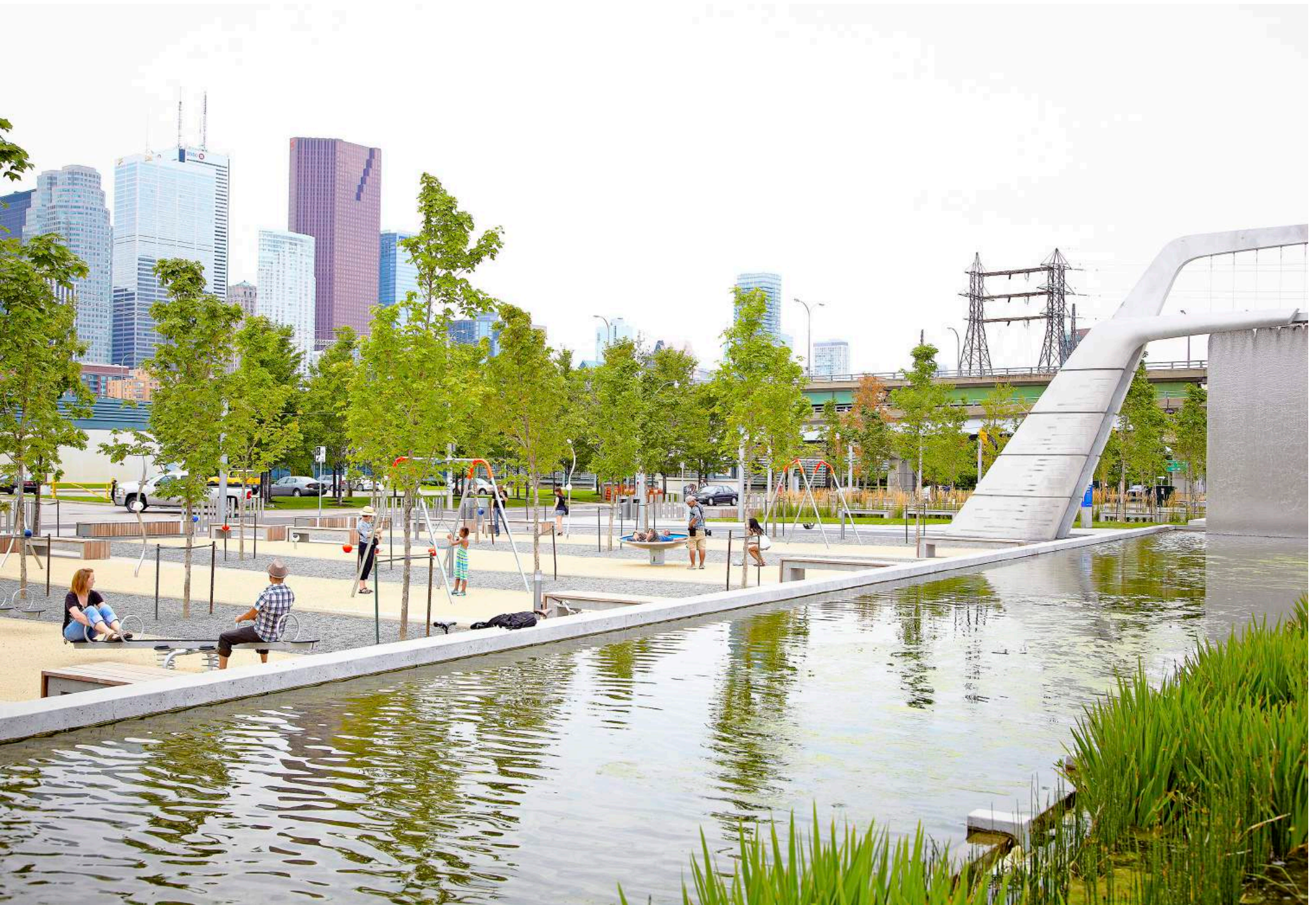
Figure 7.4 Sherbourne Commons, stormwater management system that is integrated into the park design
