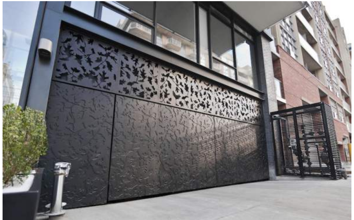
Figure 5.36 Parking and loading entrance
