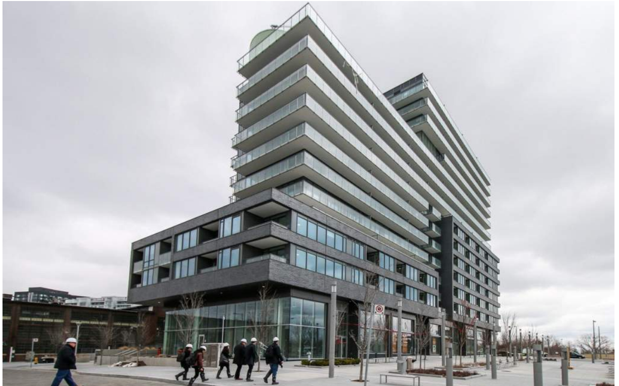
Figure 5.8 Housing in Canary District, West Don Lands (Image Credit: James Bombales)
