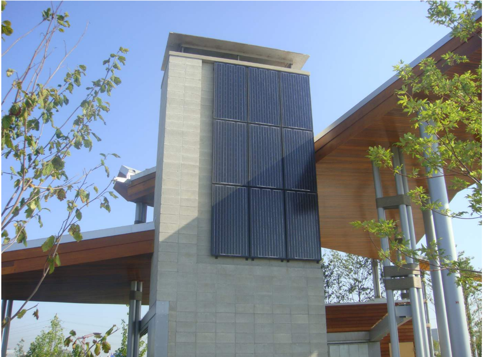
Figure 7.12 Solar Panels on washroom facility in Corktown Common
