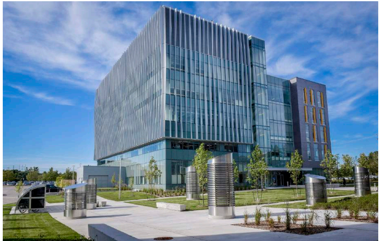
Figure 7.3 UTSC Environmental Science and Chemistry Building (LEED Gold certified) (Image Credit: UTSC)
