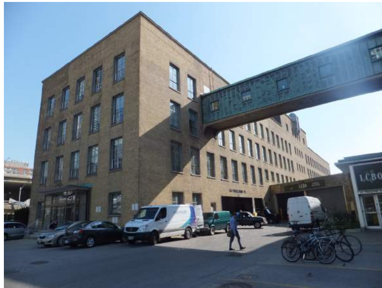
Figure 4.30 55 Lake Shore Boulevard LCBO Head Office, looking east from Freeland Street
