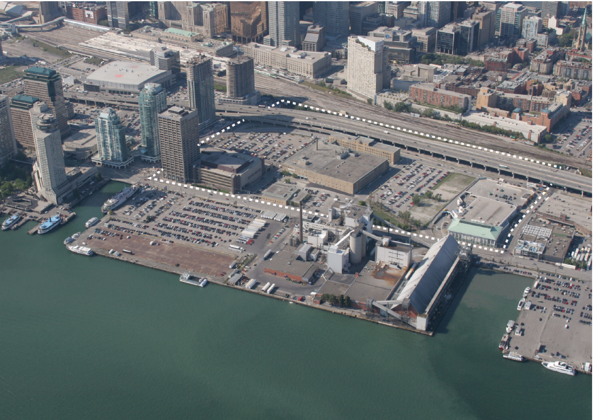
Figure 1.1 Aerial Photo of the Lower Yonge Study Area (2006)
