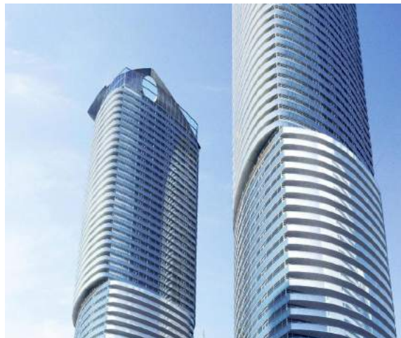
Figure 7.8 Curtain wall system, Ice Condos, Toronto (Image Credit: Urban Toronto/architectsAlliance)
