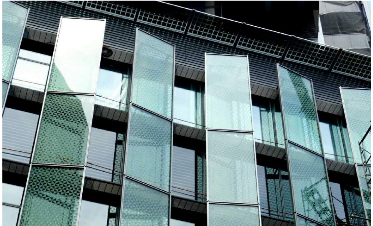
Figure 7.20 Dai Nagoya Building, Tokyo (Image Credit: Skyscraper City)
