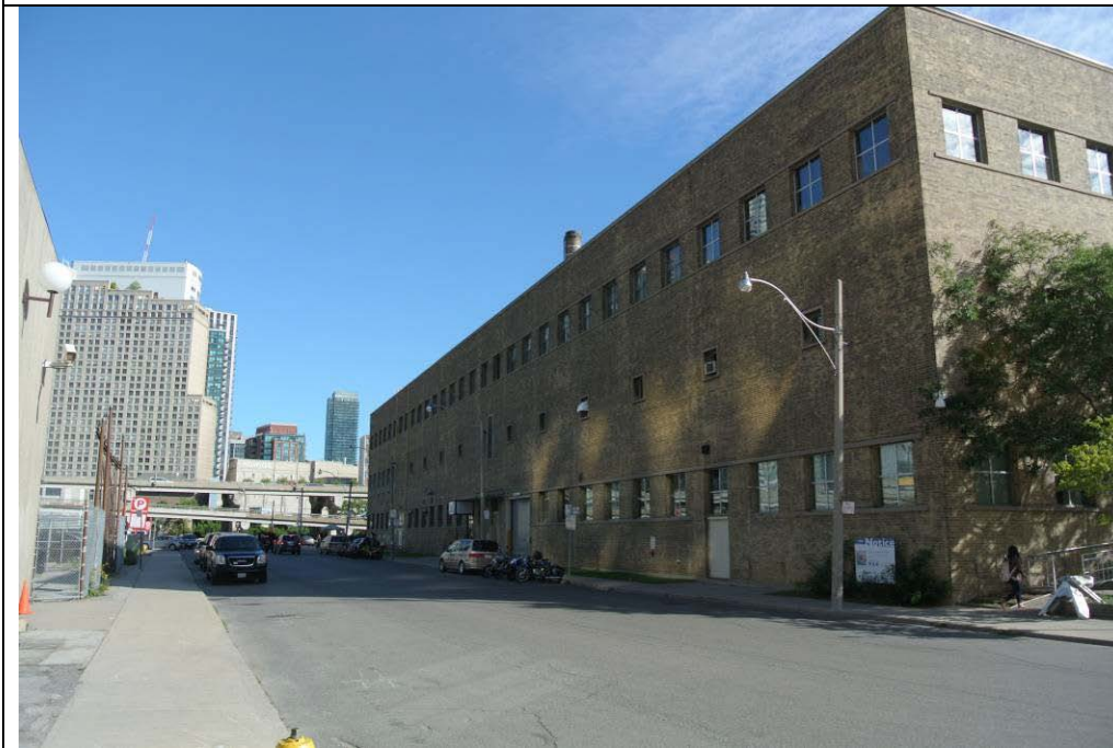
Plate 4: View north along the west elevation of the LCBO warehouse.
