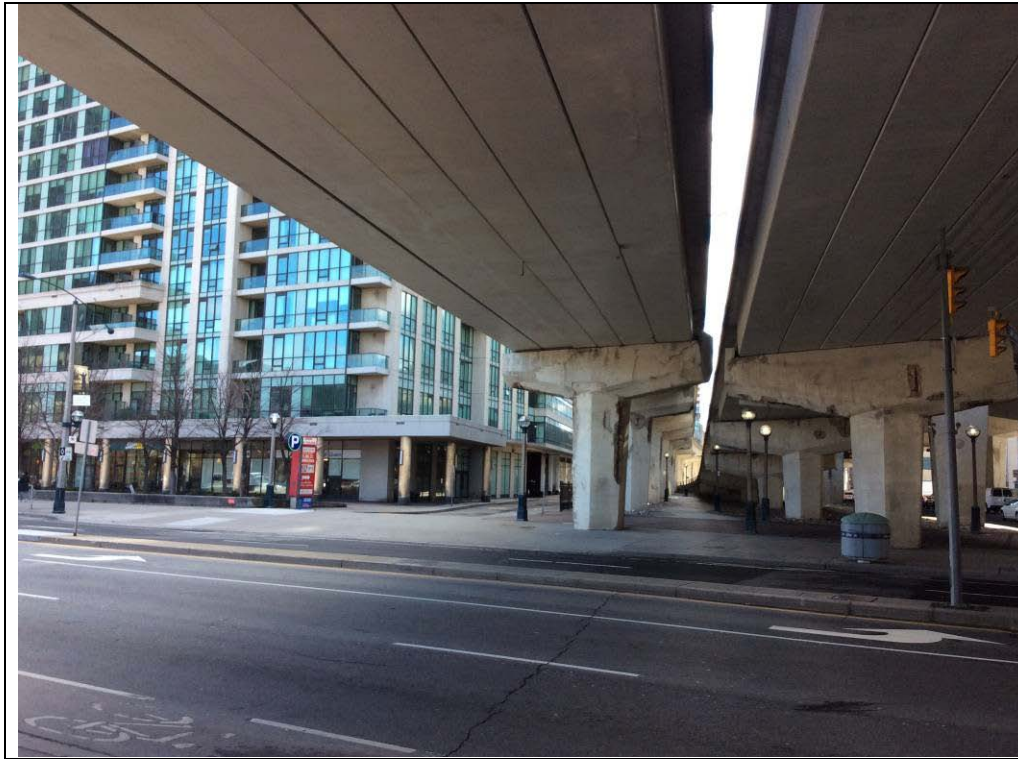
Plate 1: View west at the soffit of the Gardiner Expressway off-ramp.
