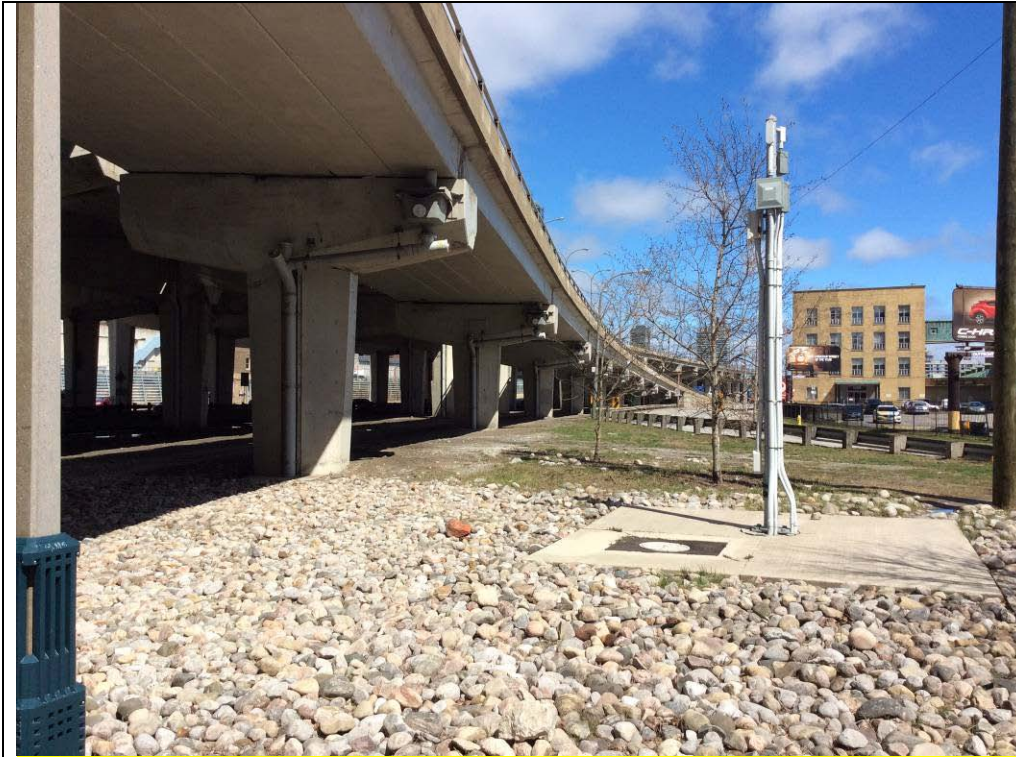
Plate 3: View west along the Gardiner Expressway off-ramp, looking east
