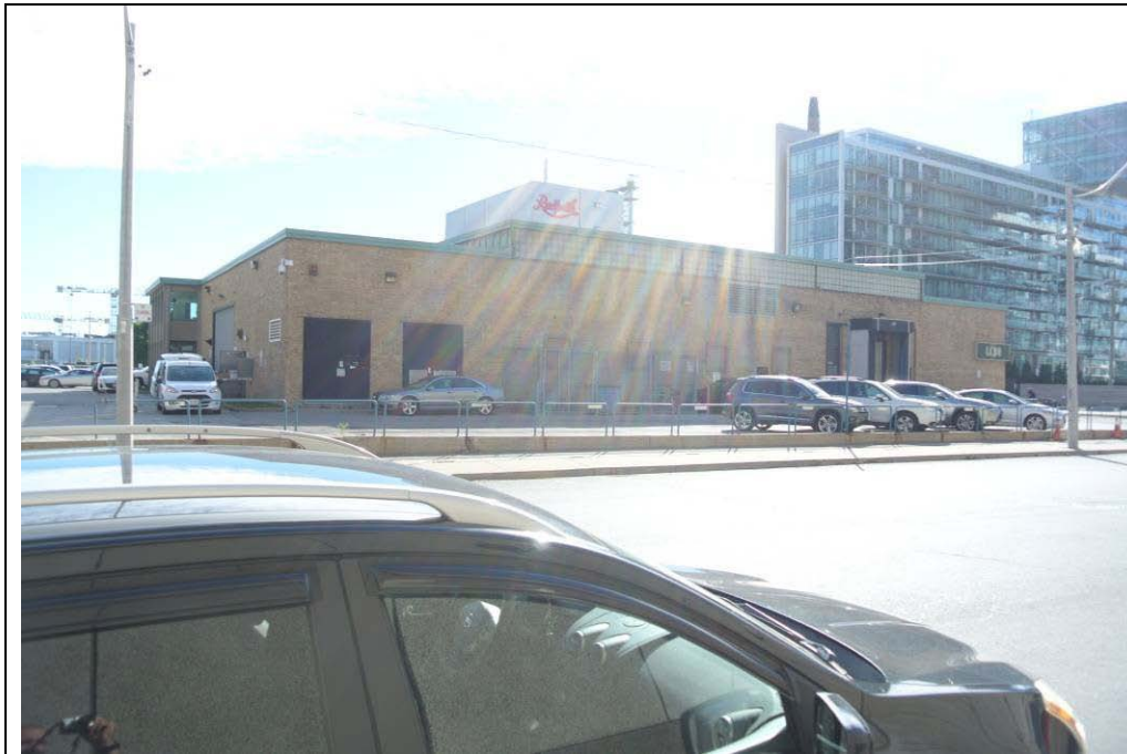
Plate 11: View southeast toward the LCBO garage and retail store.
