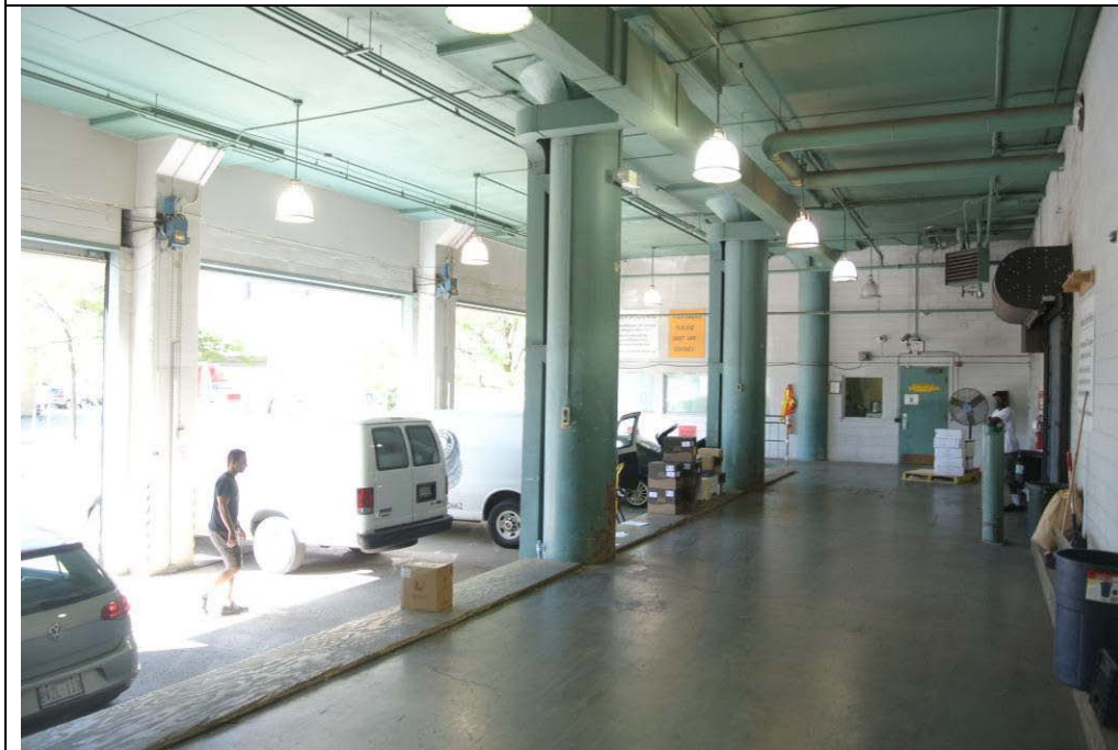
Plate 14: View of the loading docks at the south of the LCBO warehouse, looking generally west.
