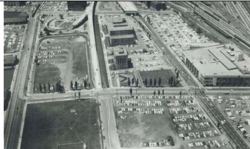
Figure 10: Construction of the Gardiner Expressway, looking west toward York Street.
