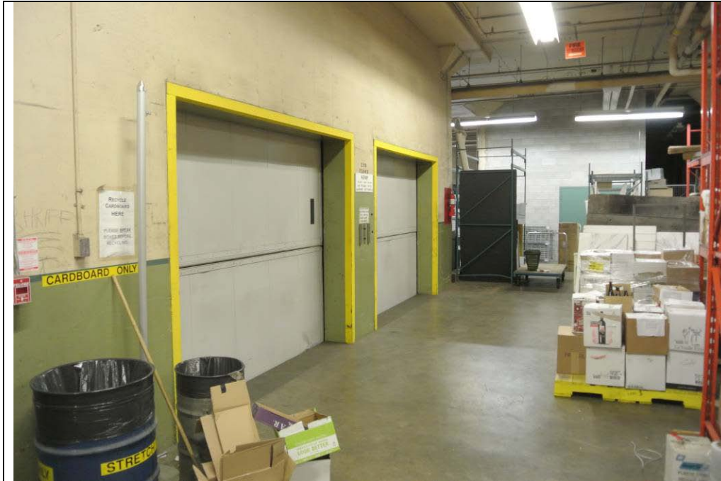
Plate 19: View toward elevators on the second floor of the LCBO warehouse.
