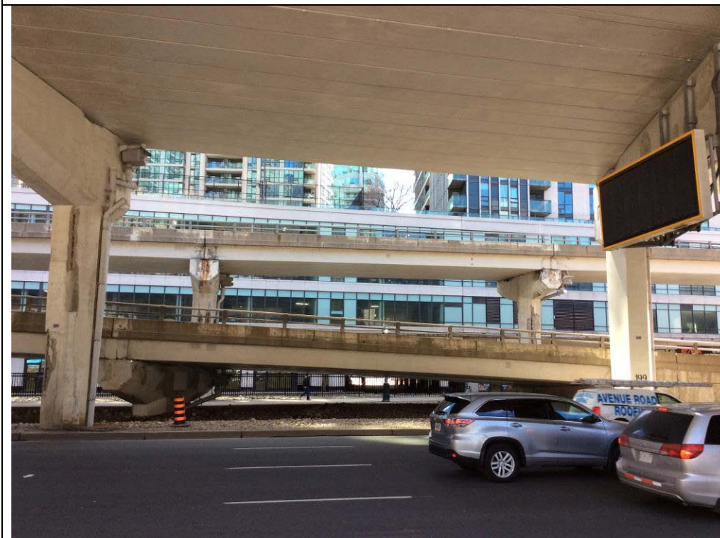
Plate 14: View south toward the Gardiner Expressway off-ramp (at back).
