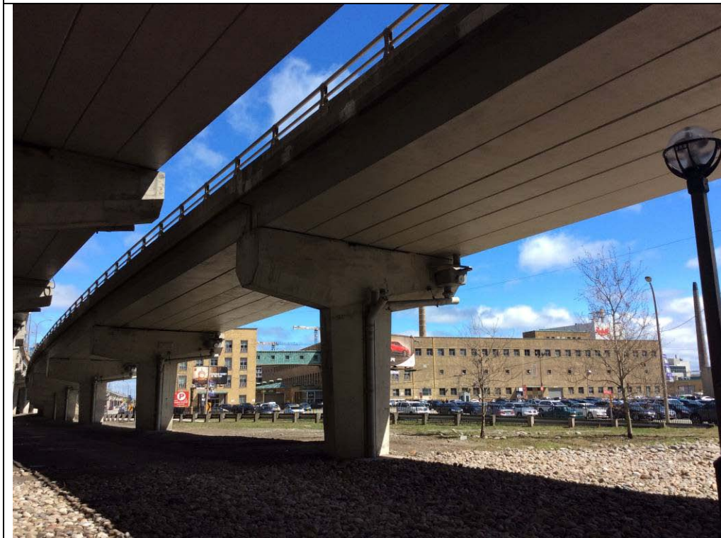
Plate 2: View east toward the soffit of the Gardiner Expressway off-ramp.
