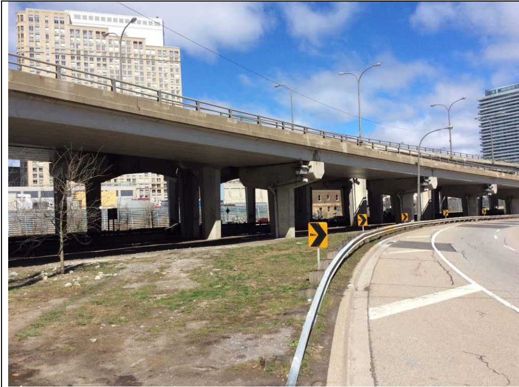
Plate 5: View northeast toward the Gardiner Expressway.
