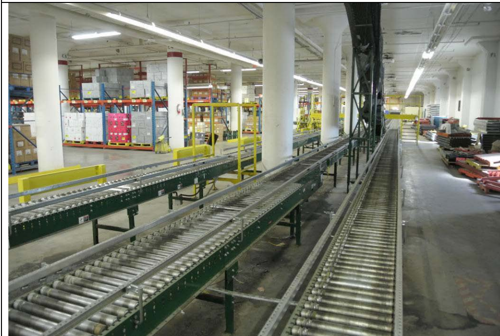
Plate 16: Detail of conveyor belt located on the second floor of the LCBO warehouse, looking generally north.
