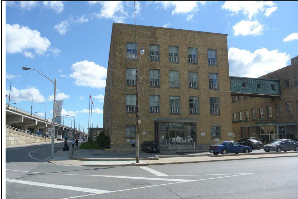
Plate 1: View east toward the LCBO office building.
