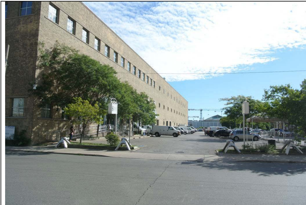
Plate 5: View east providing an oblique view of the south elevation of the LCBO warehouse.
