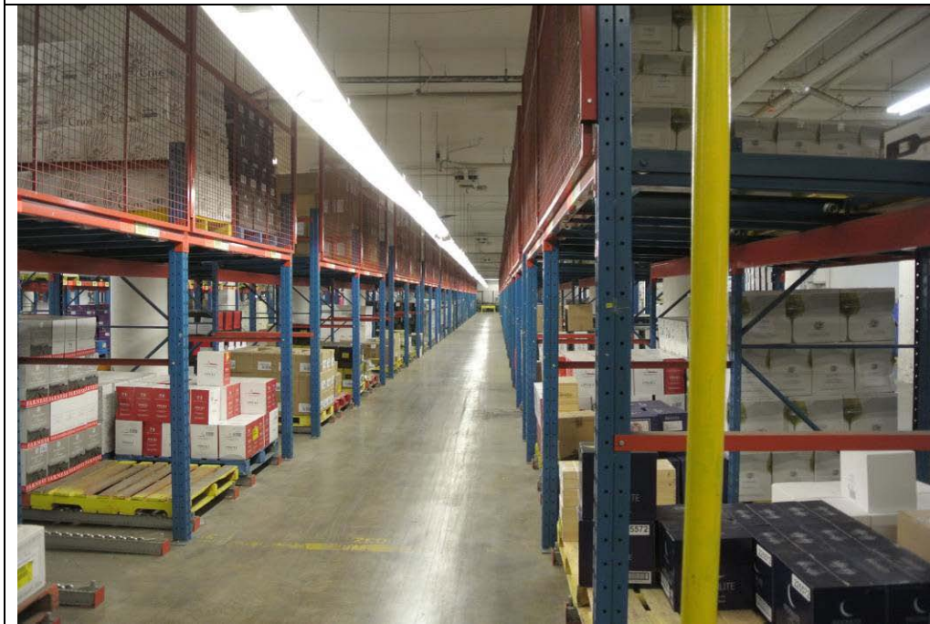
Plate 18: View of the second floor of the LCBO warehouse, looking generally east.
