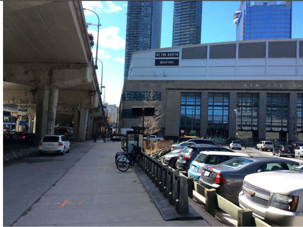
Plate 15: View of environs north of the Gardiner Expressway, looking west.
