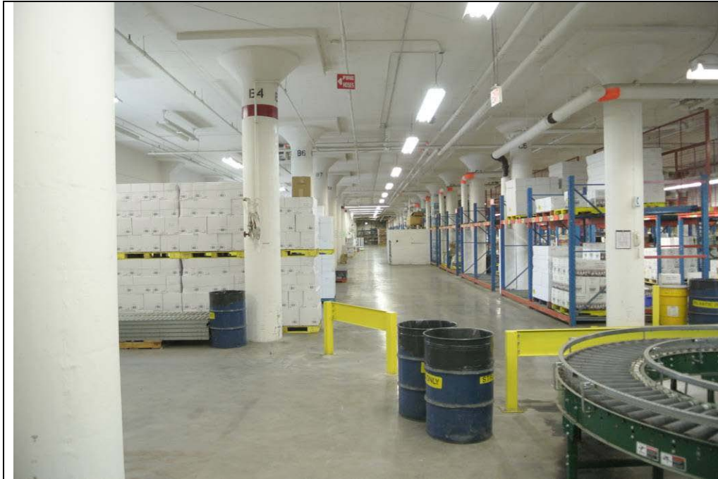
Plate 17: View of the second floor of the LCBO warehouse, looking generally west.
