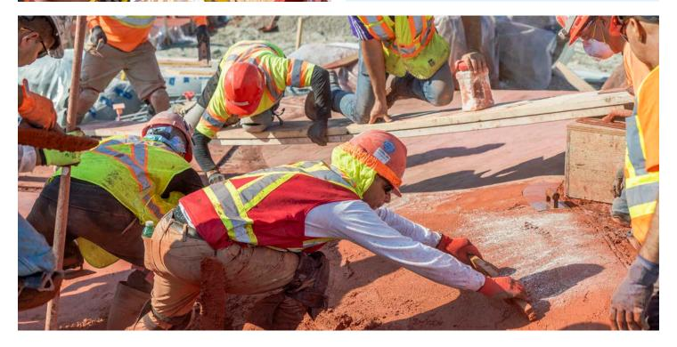
Top left: Carved beavers atop a "dam" where kids can play. Middle and right: Constructing and installing the owl and raccoon play structures. Bottom: The Badlands Scramble is constructed using spray concrete that creates an undulating, rocklike surface.
